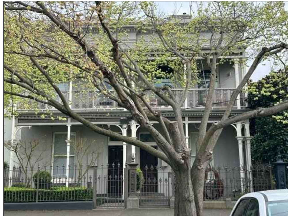
64 & 62 ST VINCENT PLACE NORTH
