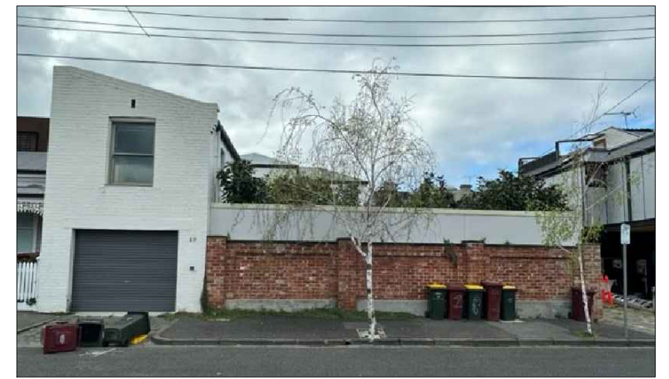
PROJECT SITE 60 ST VINCENTS PLACE NORTH REAR ELEVATION OF SITE TO DRAPER STREET
