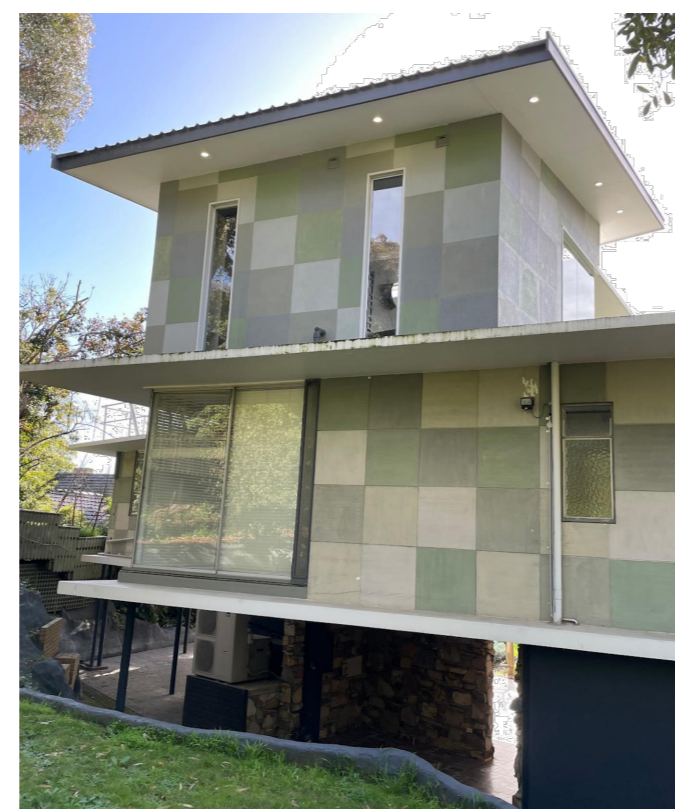
PHOTO: EXISTING HOUSE SHOWING SQUARE PANEL WALL CLADDING
