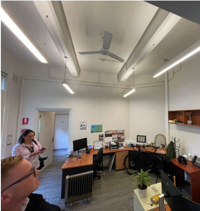
Figure 16 Ground floor office space in the location of the proposed lift core.
