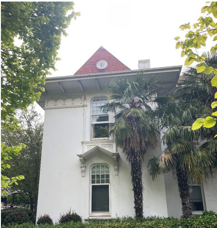
Figure 10 View of the northern end of the west elevation.
