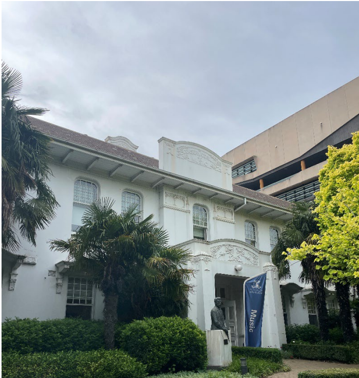
Figure 8 Exterior view of the west elevation – front of building.
