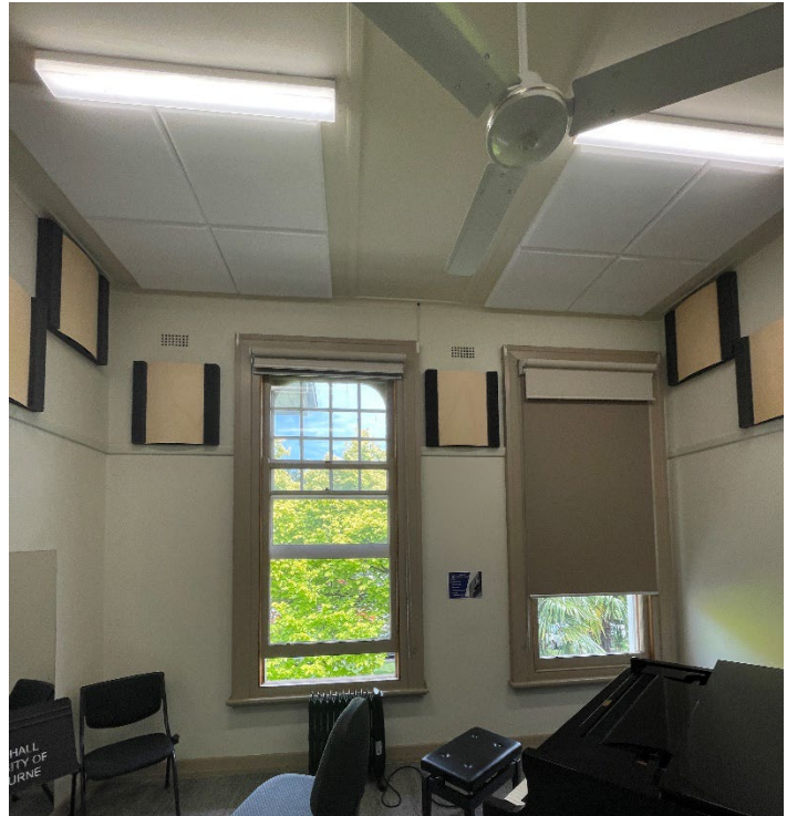
Figure 13 Typical first floor practice room showing applied acoustic treatments.
