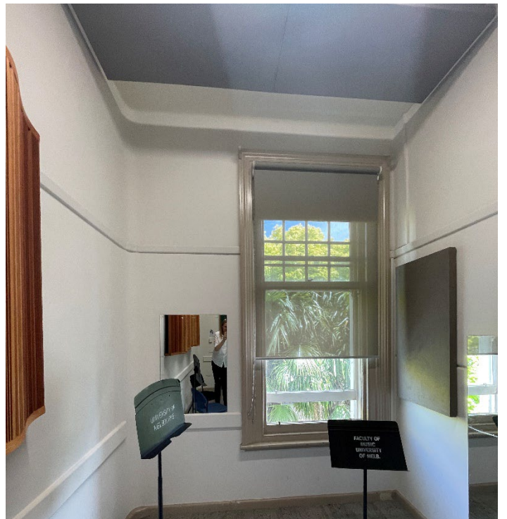
Figure 15 Typical first floor practice room showing applied acoustic treatments.
