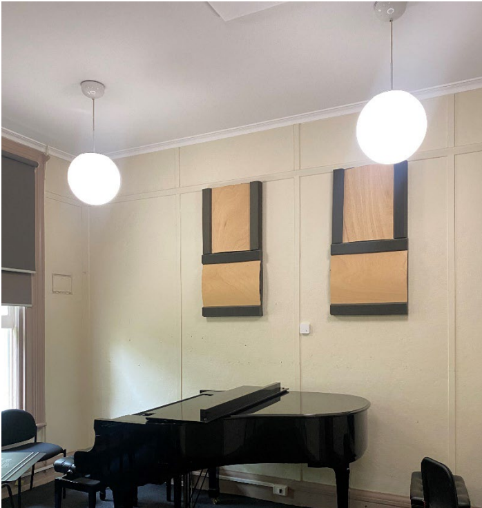
Figure 12 Typical first floor practice room showing applied acoustic treatments.
