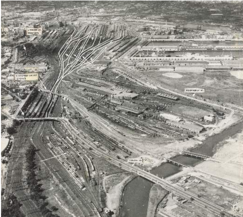
Figure 182 Aerial photograph looking south over North Melbourne Railway Station, showing goods yard, Spencer Street station. Evident are Melbourne Goods Yard alterations, c.1962 (Source: SLV, Record ID: 9923973633607636)
