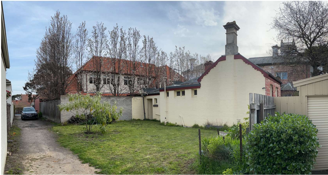
Figure 5: Subject site, east view off the rear lane. The 1890's cottage with rendered masonry chimney is to the right. The contemporary flat roof addition is to the left in matching painted brick. The east facade of the two-storey villa is visible in the background.
