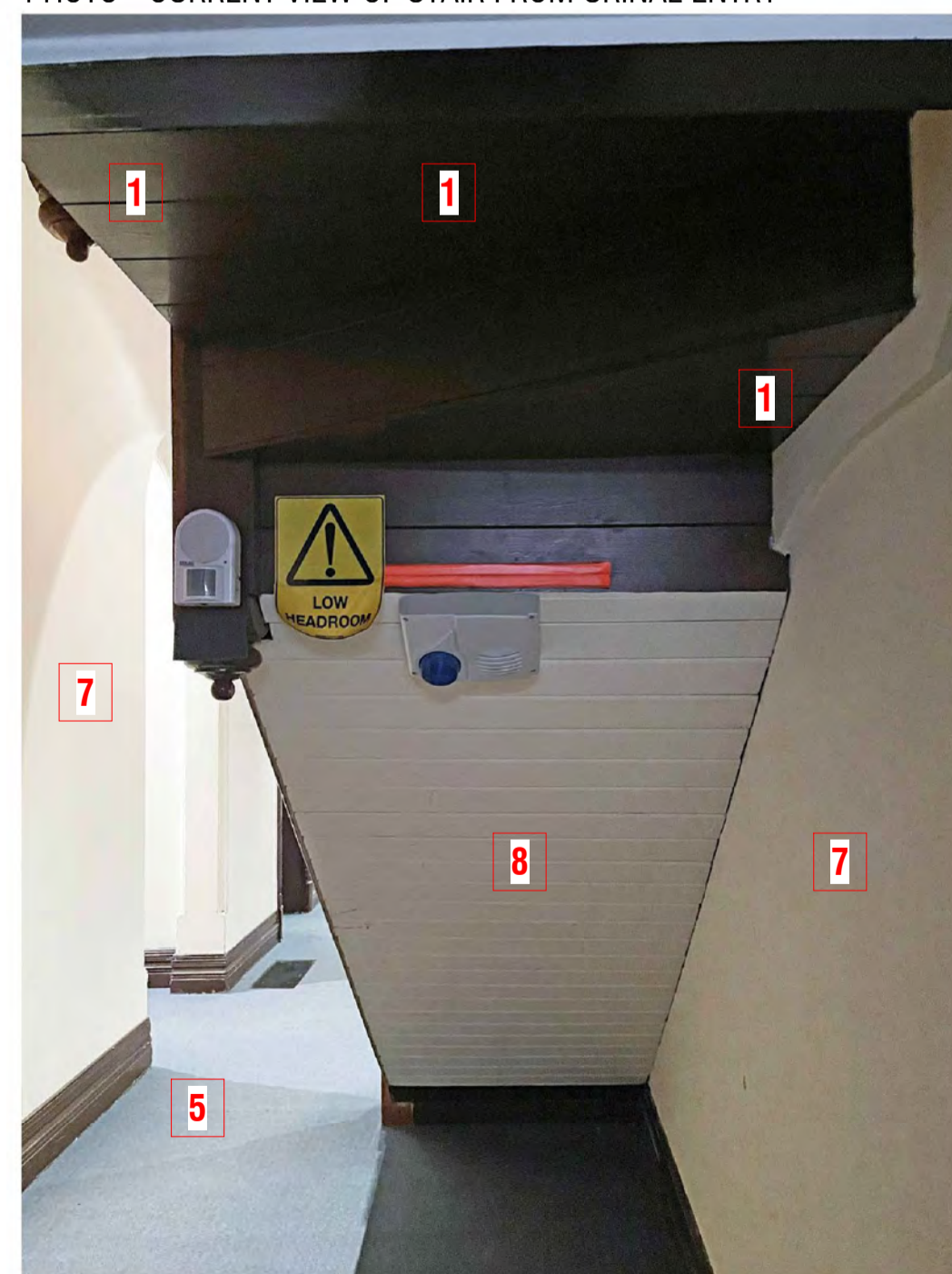
PHOTO - CURRENT VIEW OF STAIR FROM URINAL ENTRY
