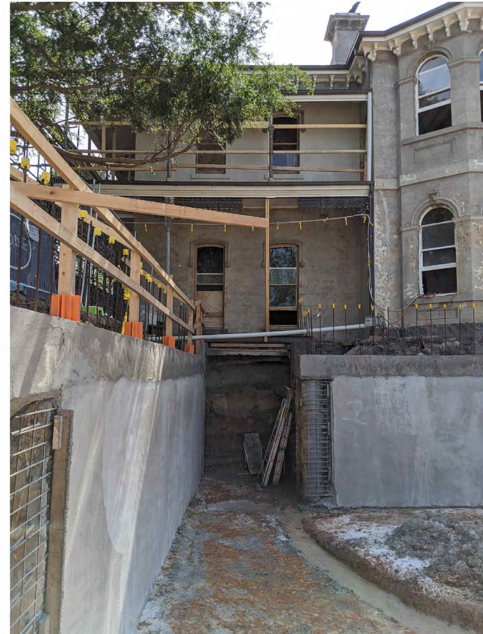
REFERENCE PHOTO - SHOTCRETE WALL SPRAYED TO BASEMENT AFTER EXCAVATION COMPLETED
