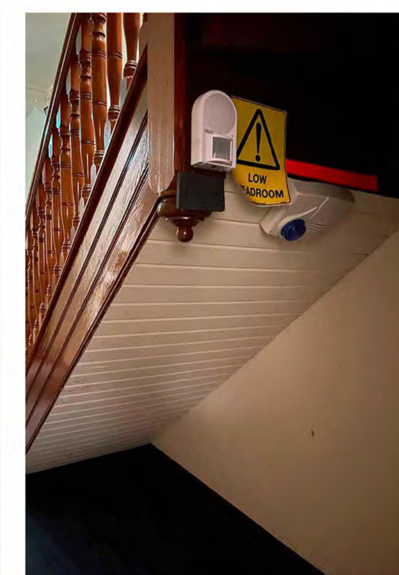
SITE PHOTO #2 • EXISTING LOW HEADROOM CLEARANCE UNDER STAIR
