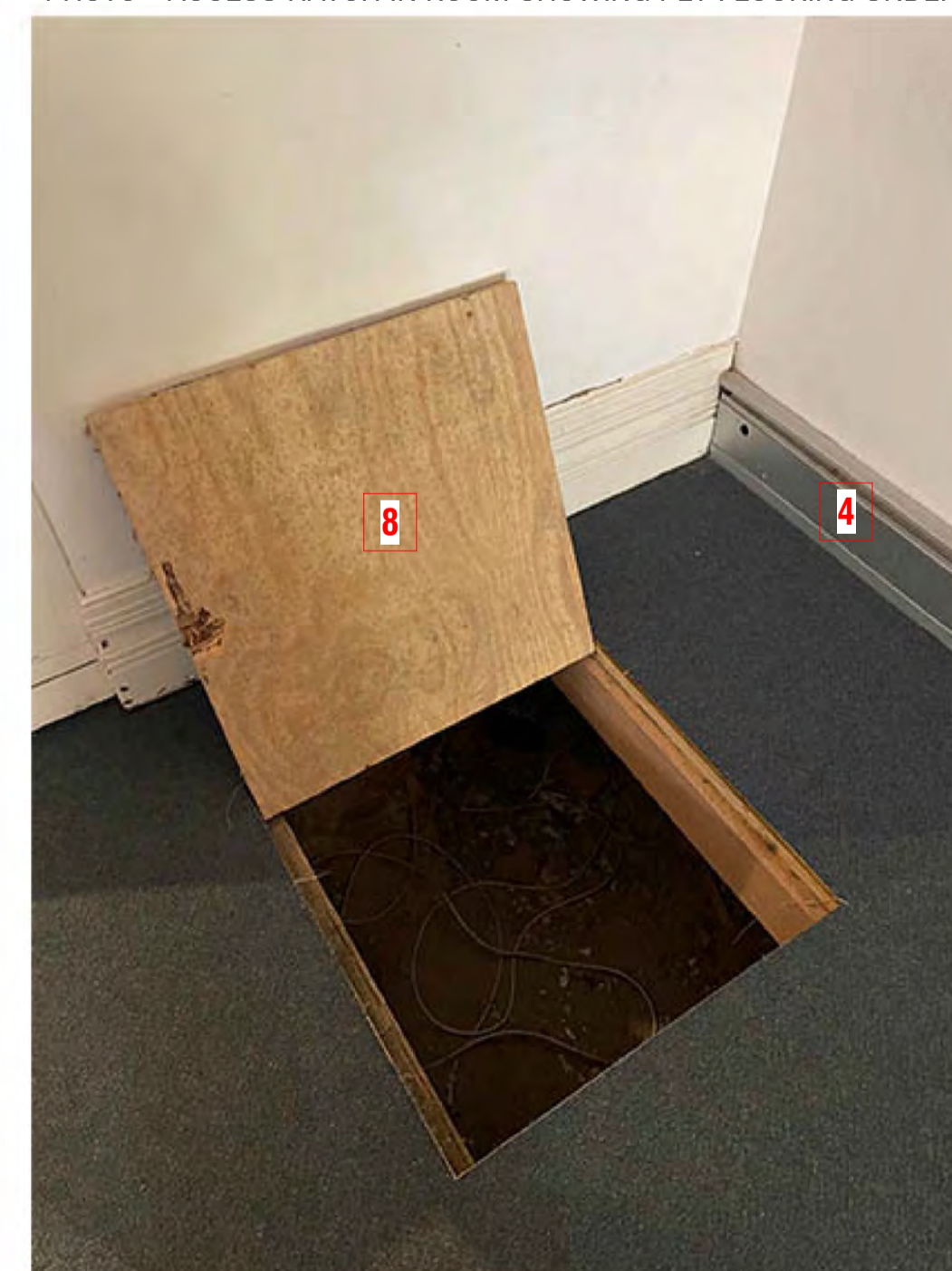
PHOTO - ACCESS HATCH IN ROOM SHOWING PLY FLOORING UNDER
