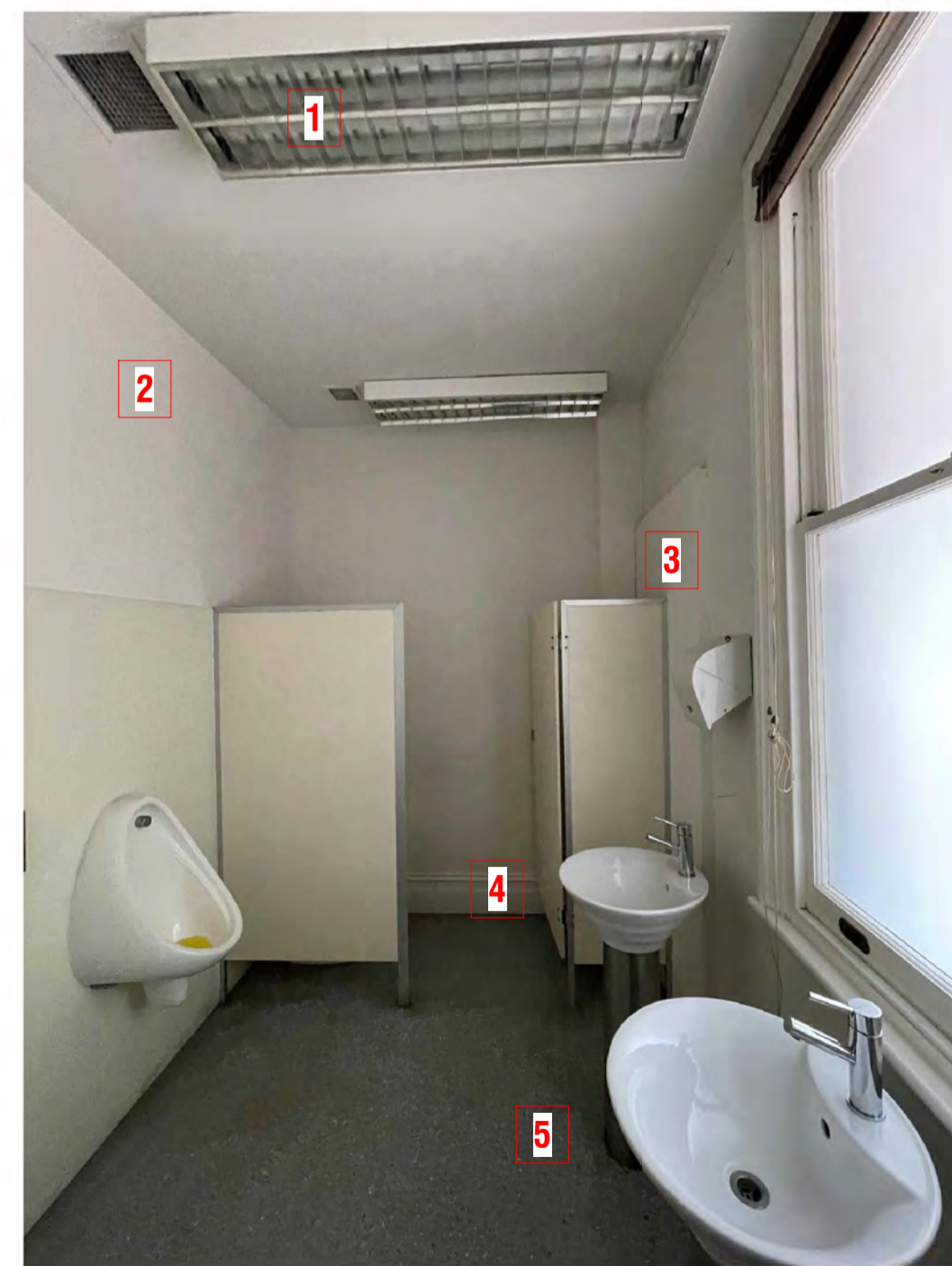
PHOTO - CURRENT VIEW INTO URINAL
