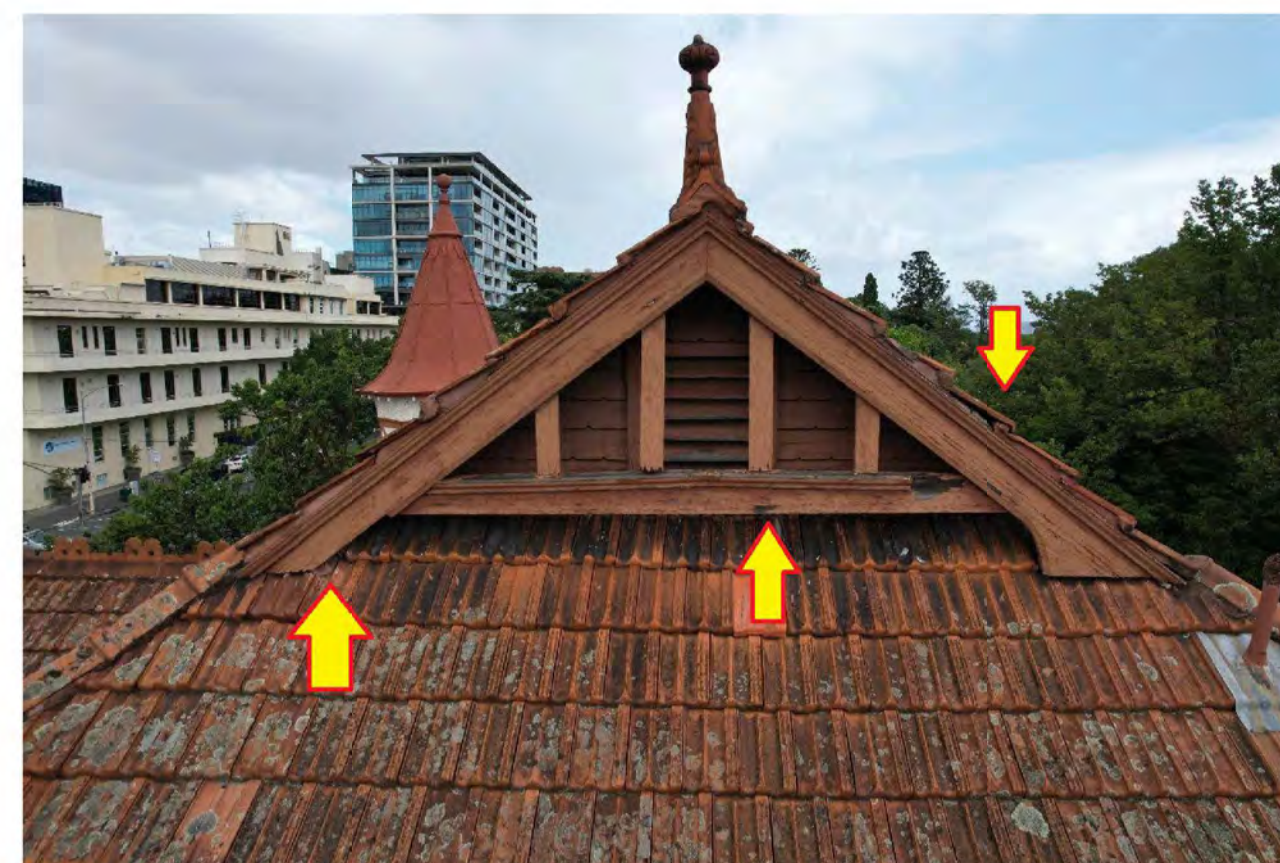
ROTTEN TIMBER AND DILAPIDATED
