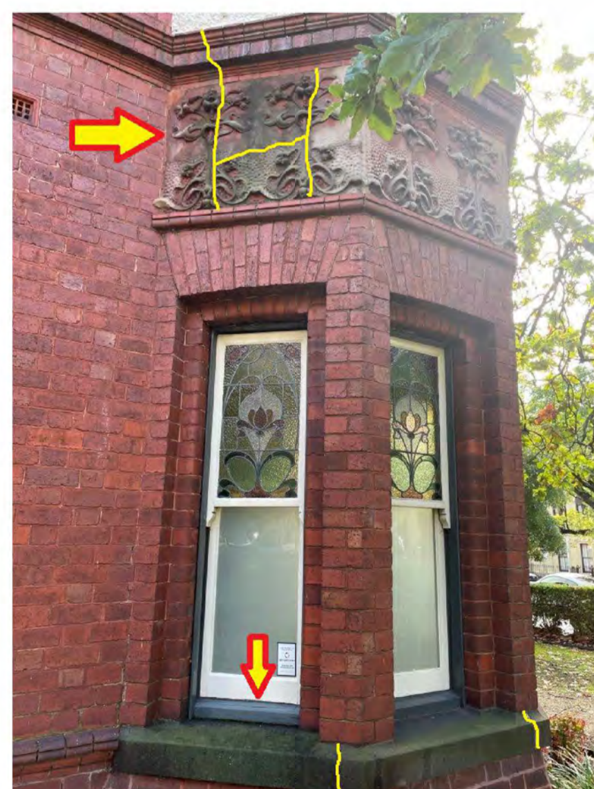
WATER DAMAGE BEHIND TERRACOTTA TILES. ROTTEN TIMBER SILLS
