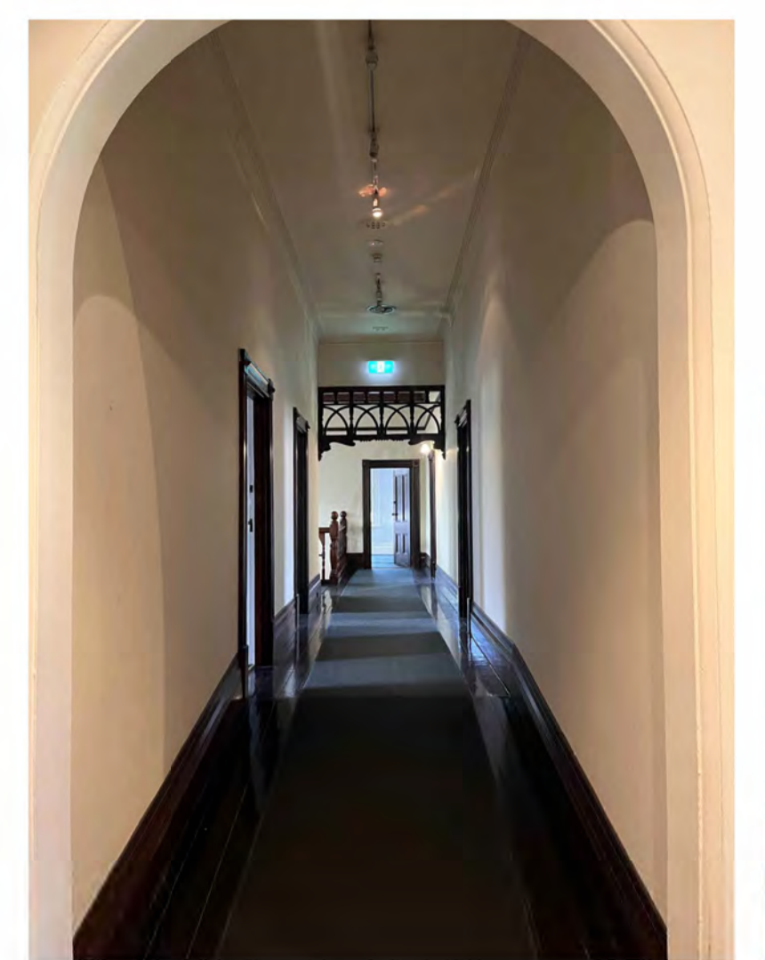
EXISTING CONDITIONS - FIRST FLOOR HALLWAY CEILING
