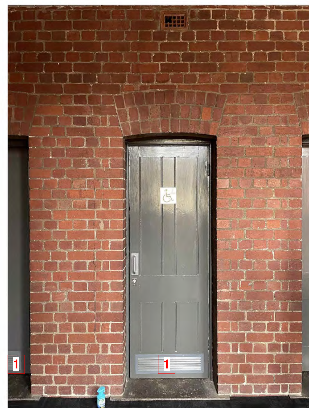
PHOTO - CURRENT WC DOORS
