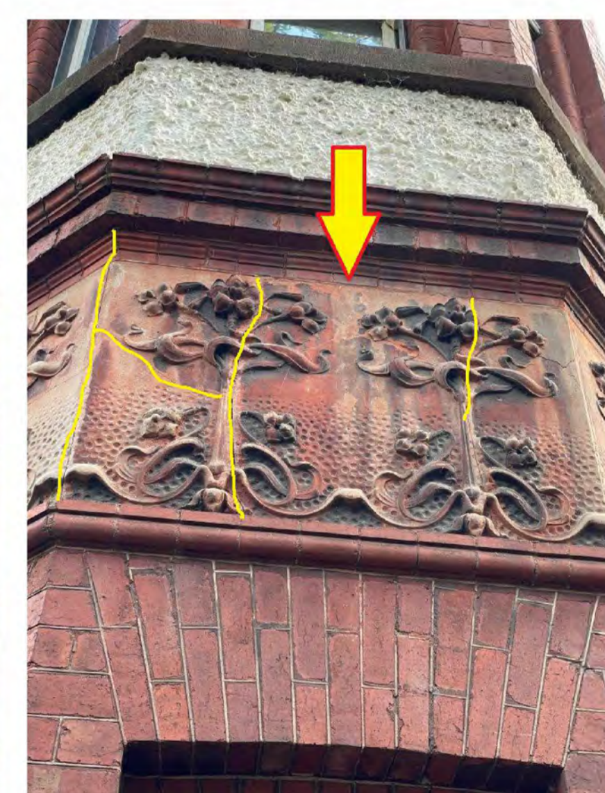
WATER DAMAGE BEHIND TERRACOTTA TILES. ROTTEN TIMBER SILLS
