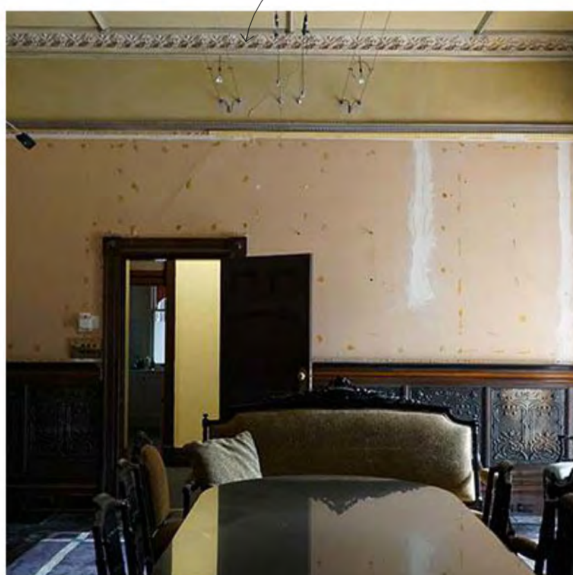
ROOM: MEETING ROOM 02 CORNICE: ORIGINAL CORNICE
