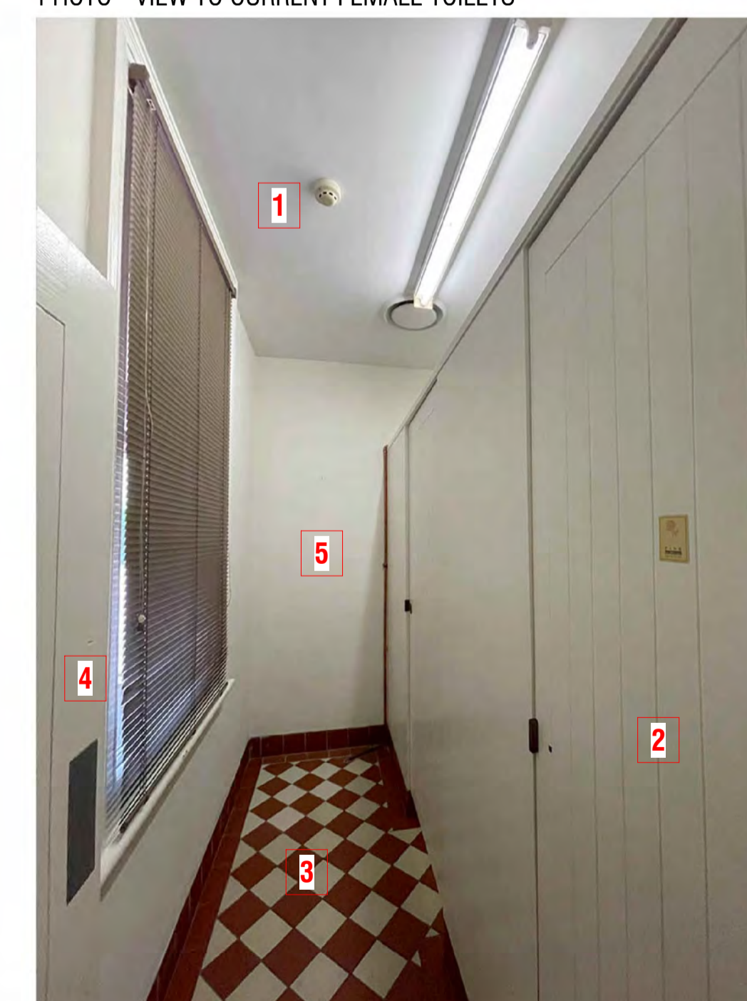
PHOTO - VIEW TO CURRENT FEMALE TOILETS
