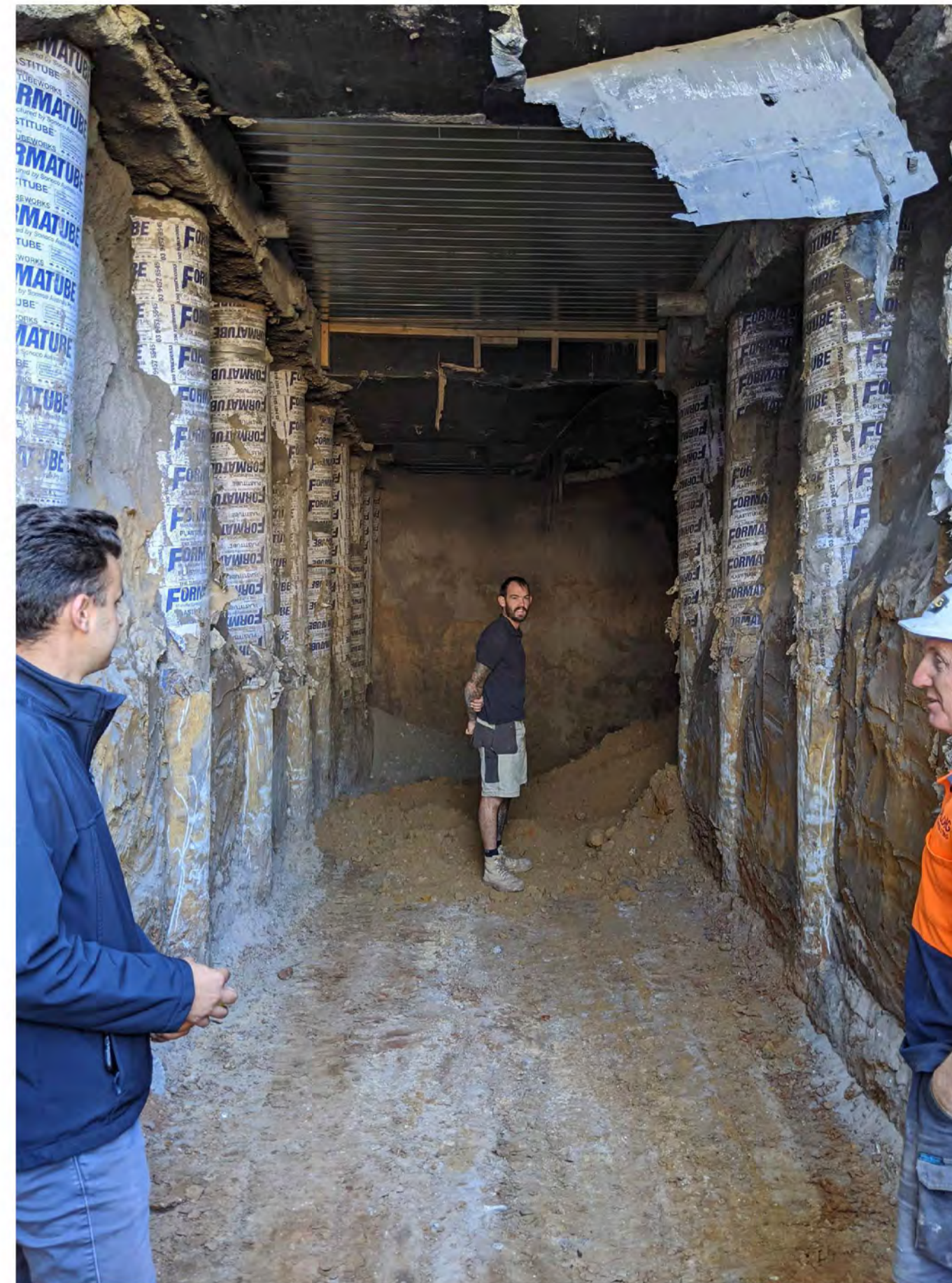
REFERENCE IMAGE - TOP DOWN CONSTRUCTION BORED PILES CONSTRUCTED WITH CAPPING BEAM AND GROUND FLOOR SLAB SPANING BETWEEN FOR BRACING
