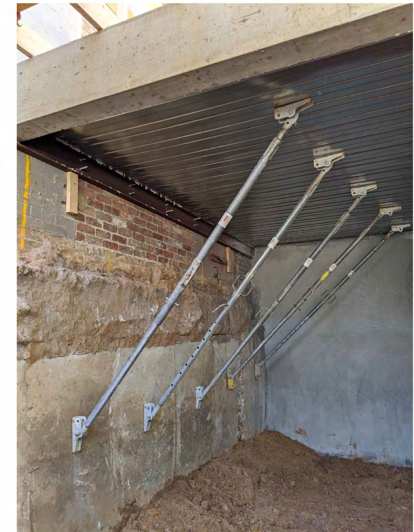
REFERENCE IMAGE - GROUND FLOOR SLAB PROPPED TO BASEMENT DURING EXCAVATION
