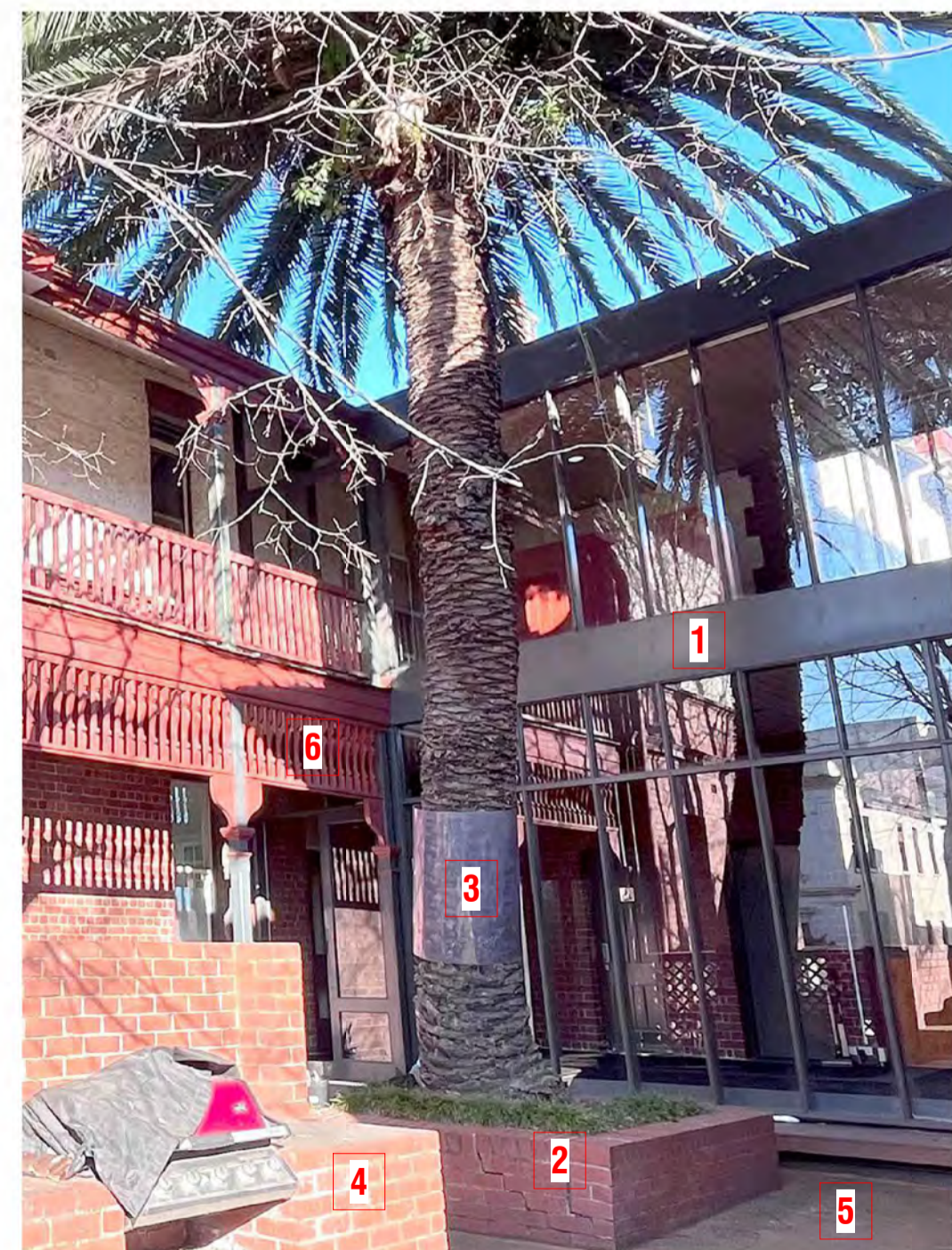
PHOTO - VIEW TOWARDS CURRENT BUILDING LINK
