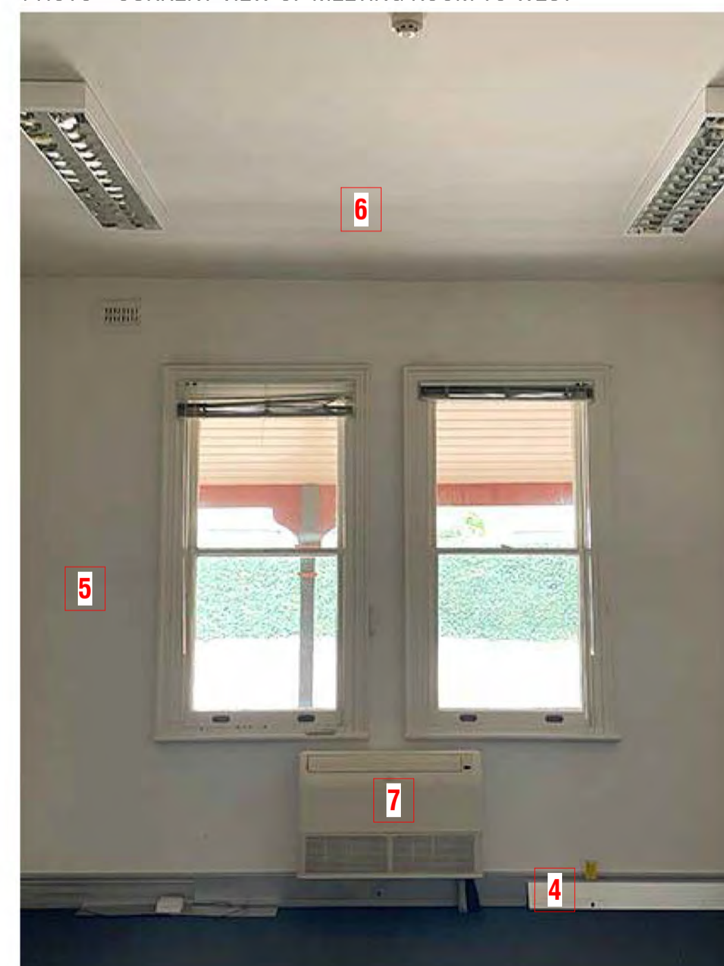
PHOTO - CURRENT VIEW OF MEETING ROOM TO WEST
