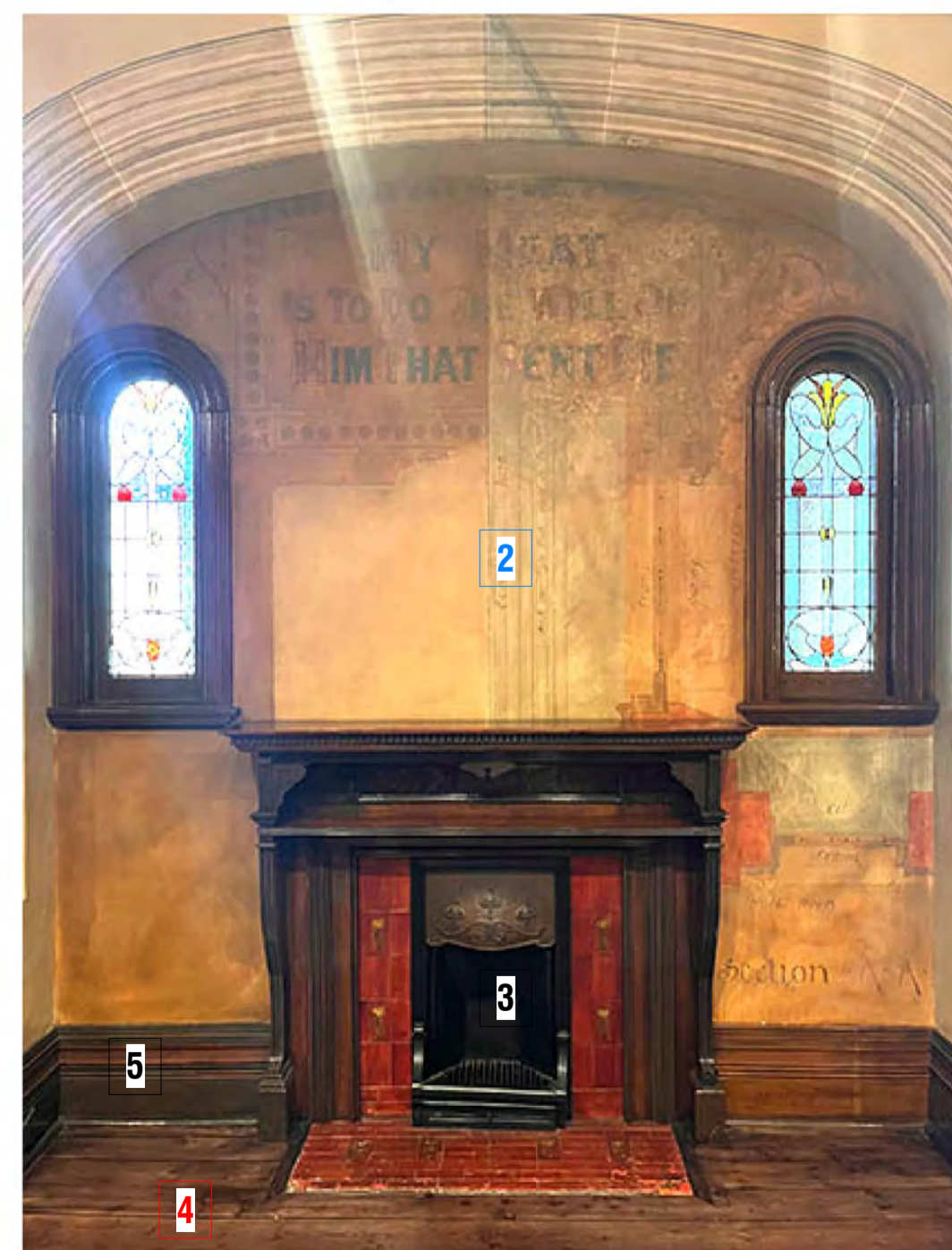
PHOTO - CURRENT VIEW CLOSE-UP OF ALCOVE
