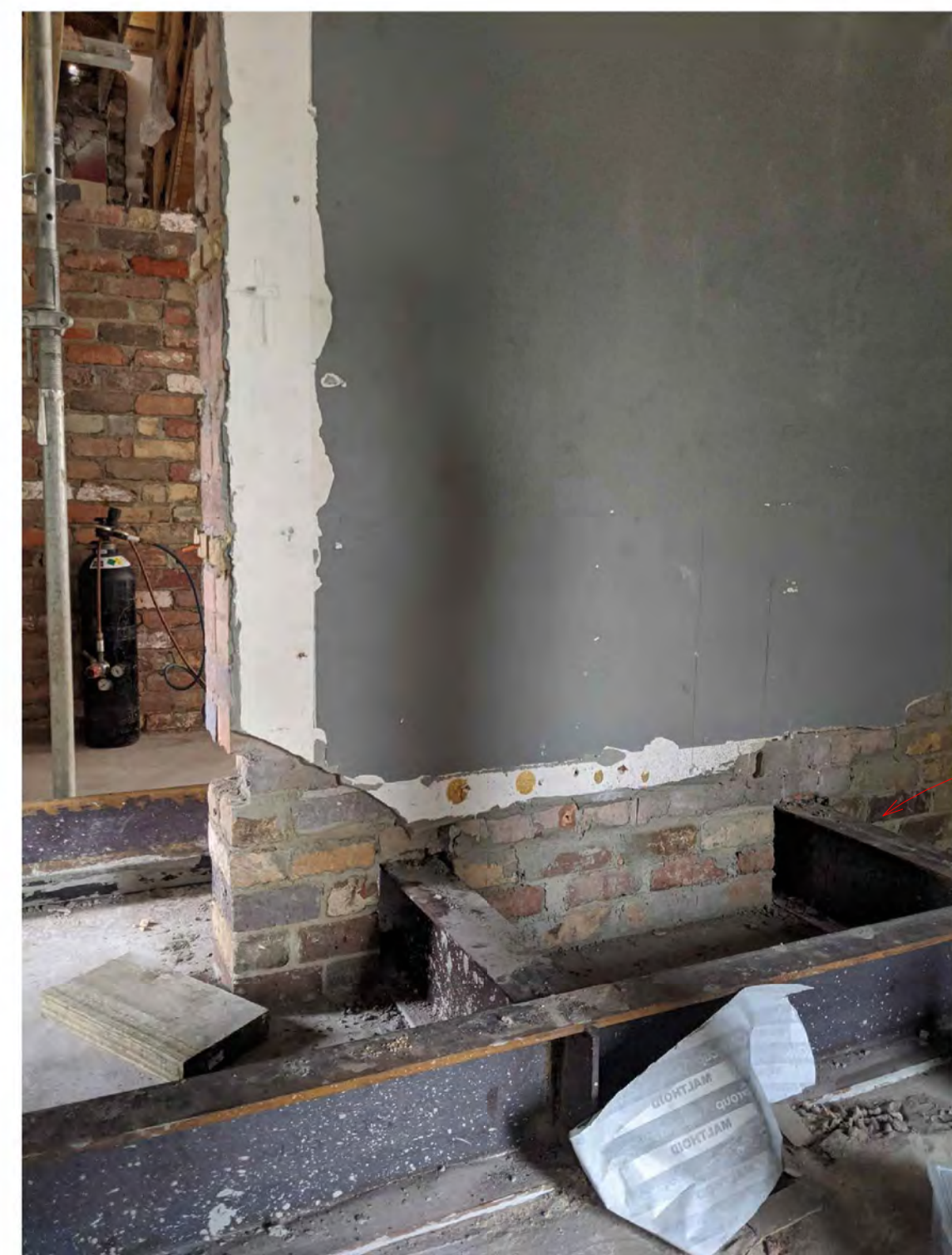
REFERENCE IMAGE - HERITAGE WALLS TEMPORARILY PROPPED USING NEEDLING TECHNIQUES AT GROUND LEVEL
