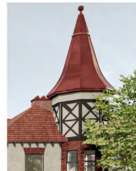
TIMBER DECORATIVE STRAPPING CHECK TIMBER FOR DECAY, REPAIR AND TREAT ROT. PAINT RESENE 'IRONSAND' OR SIMILAR
