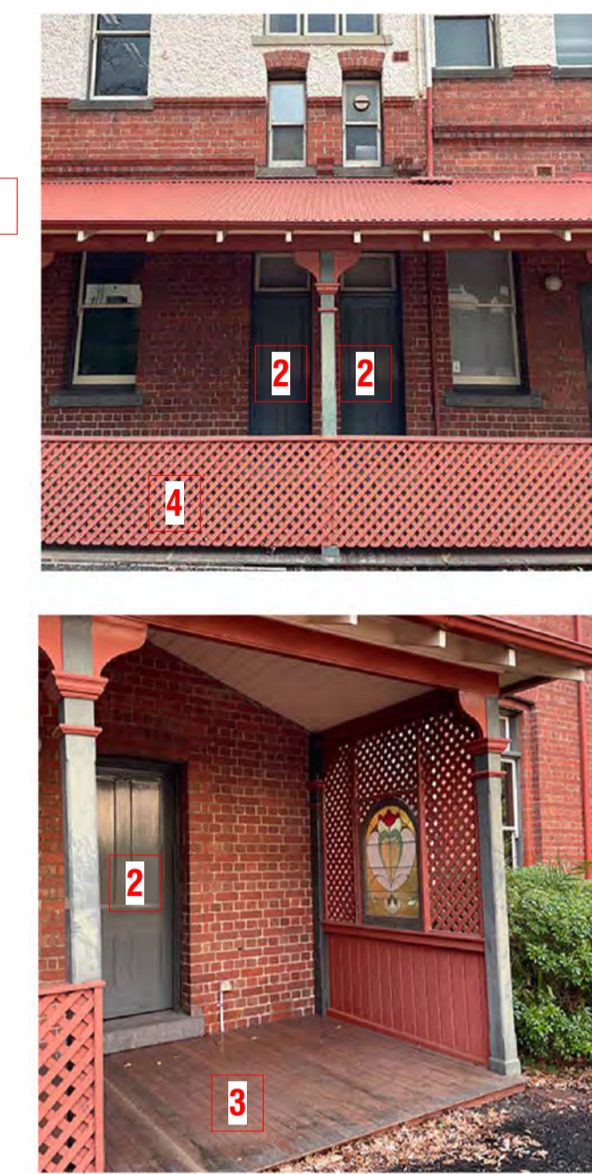
PHOTO - CURRENT VIEW OF EXTERNAL VERANDAH
