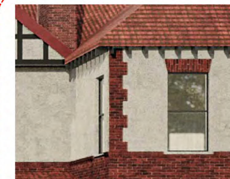
WINDOW FRAMES & GLASS MAKE GOOD EXISTING WINDOW FRAME, TREAT DECAY TIMBER FRAME PAINTED WITH RESENE 'IRONSAND' OR SIMILAR REPAIR MECHANISMS, CORD, WINDOW SEAL TO MAKE WINDOWS OPERABLE AND SMOOTH. REPLACE SINGLE FLOAT GLASS WITH LAMINATED SAFETY GLASS FOR CODE COMPLIANCE
