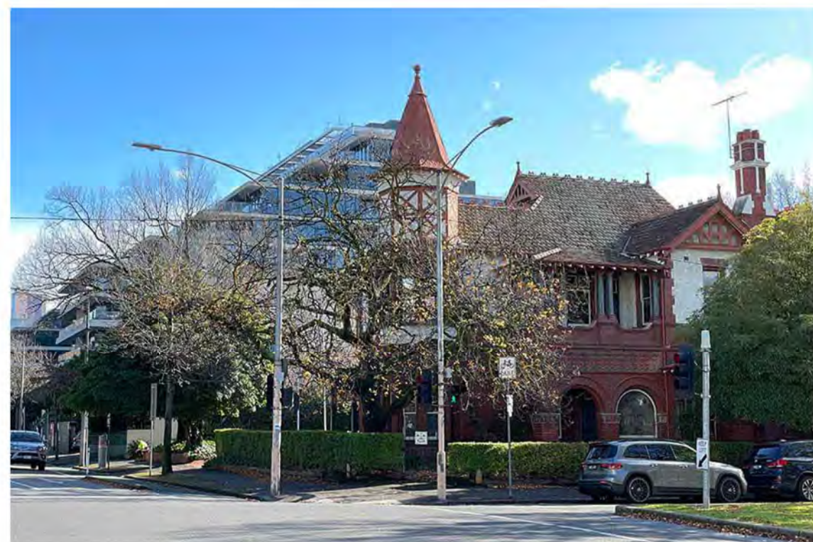
CLARENDON/ ALBERT ST VIEW - FROM CORNER
