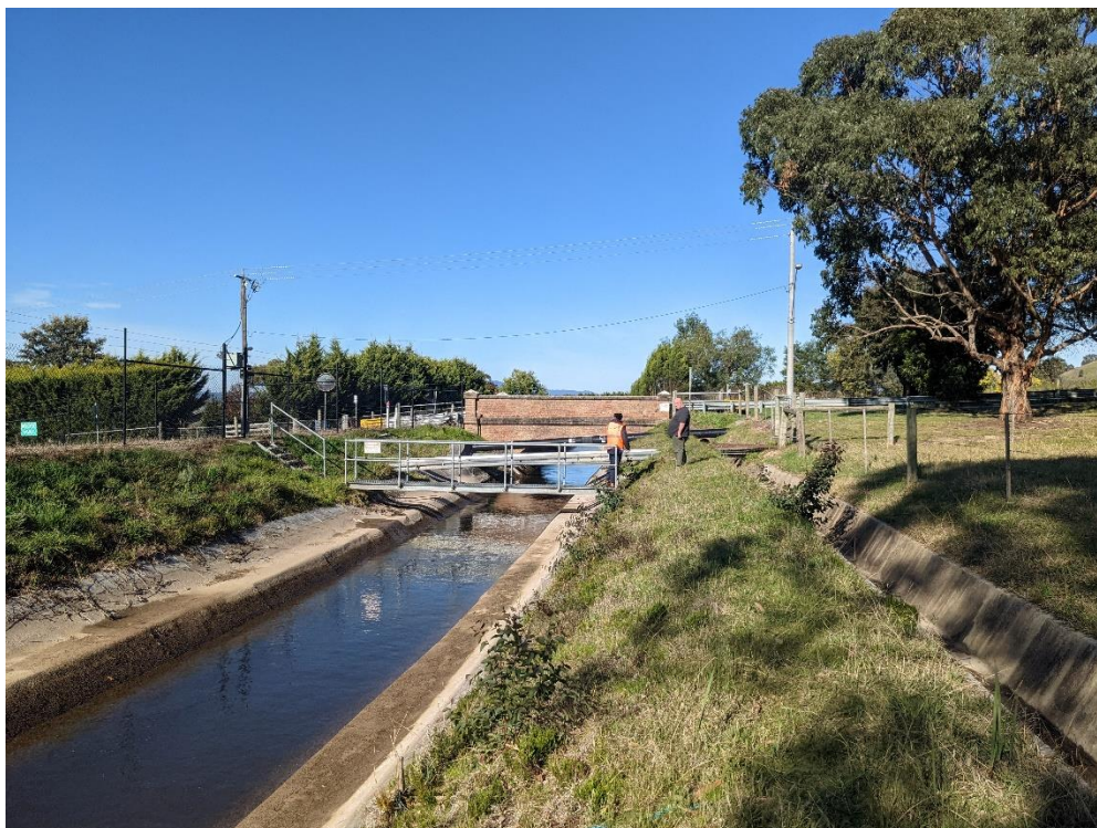
Figure 4.5 View of the northern side of the bridge. (Source: GML August 2023)
