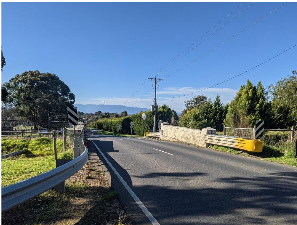
Figure 4.1 Eastern approach to the Eltham-Yarra Glen Road bridge. (Source: GML August 2023)
