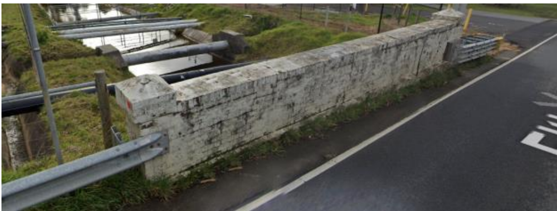
Figure 5.4 Existing safety barriers to be removed during construction (north side) (source: DTP)
