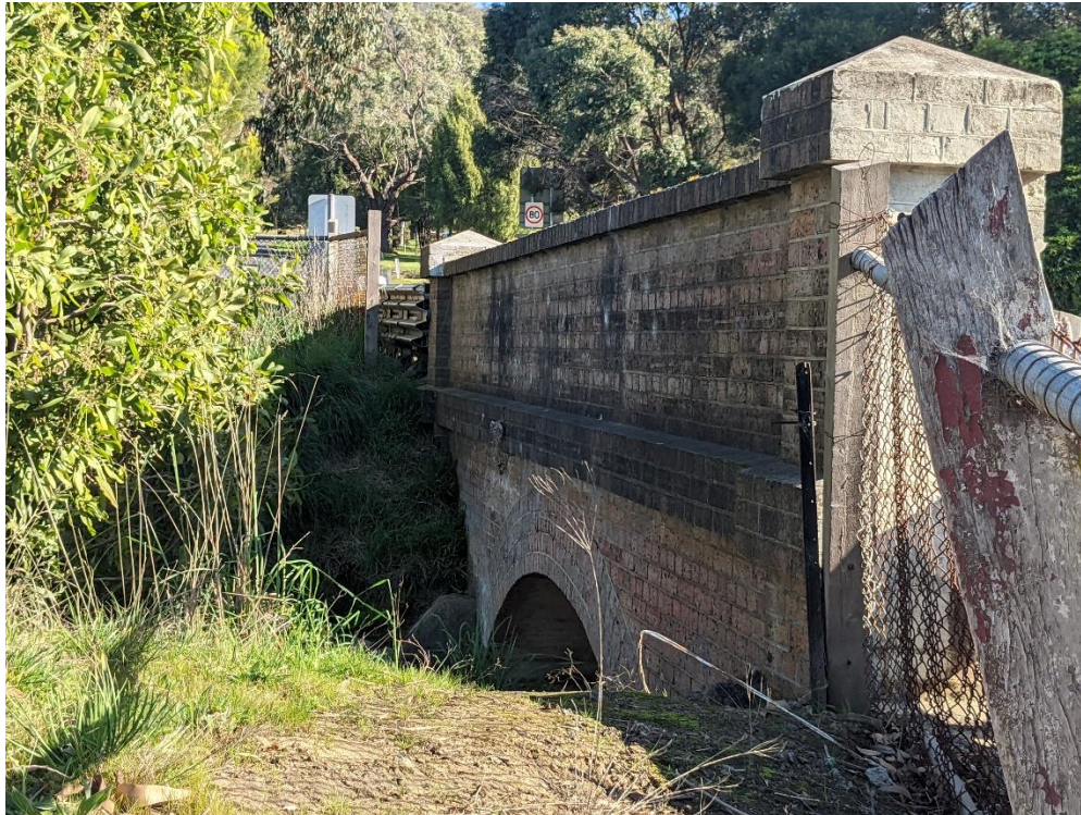
Figure 4.8 View of the southern side of the bridge. (Source: GML August 2023)
