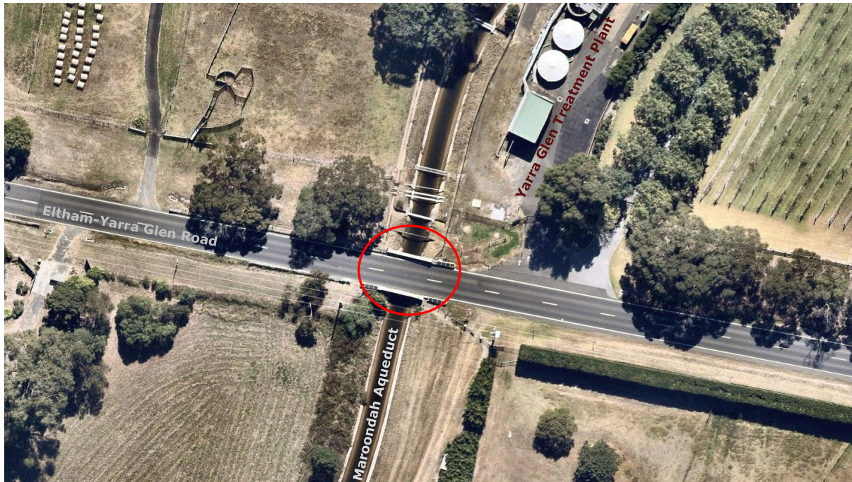
Figure 1.2 Aerial view of the Eltham-Yarra Glen Road bridge (denoted by red outline). Source: Nearmap April 2024, with GML overlay)
