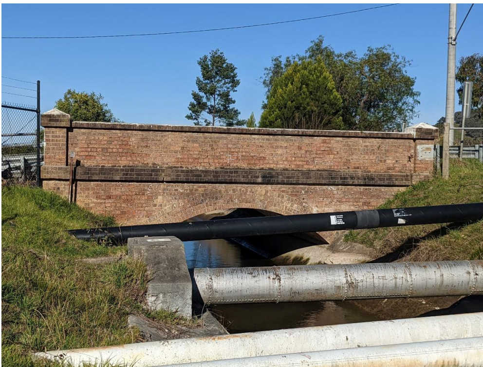
Figure 4.3 Northern side of the bridge. (Source: GML August 2023)
