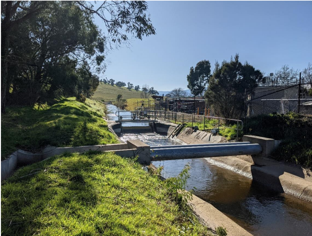
Figure 4.6 View of Maroondah Aqueduct looking north. (Source: GML August 2023)
