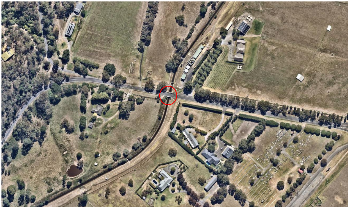
Figure 1.1 Aerial view of the Eltham-Yarra Glen Road bridge (denoted by red outline). (Source: Nearmap April 2024, with GML overlay)
