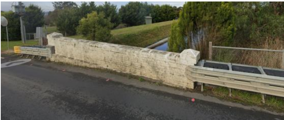
Figure 5.3 Existing safety barriers to be removed during construction (south side) (source: DTP)
