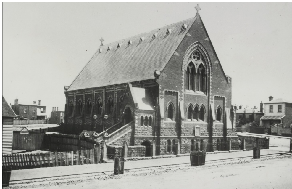
Figure 4 St Jude's Anglican Church viewed from Lygon Street, 1876 Source: State Library of Victoria .
