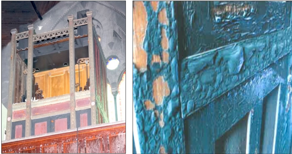
Figure 9 Photographs of the fire damaged organ, showing much of the lead pipework destroyed and blistered paintwork to the casing.
