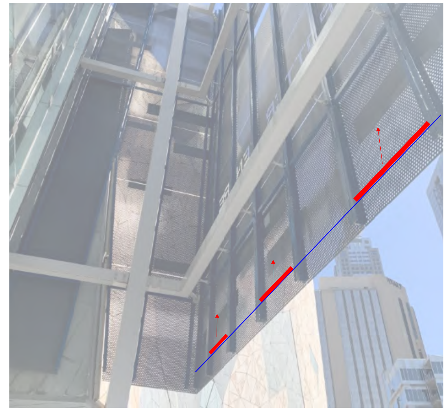
DETAIL 10 Linear light to back of the screen NTS
