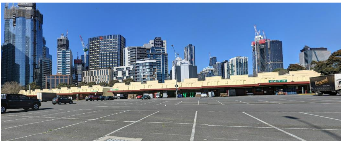
Figure 12. South-east facing view of Franklin Street Stores from the north-west corner of the carpark. Source: Extent Heritage, 2021.
