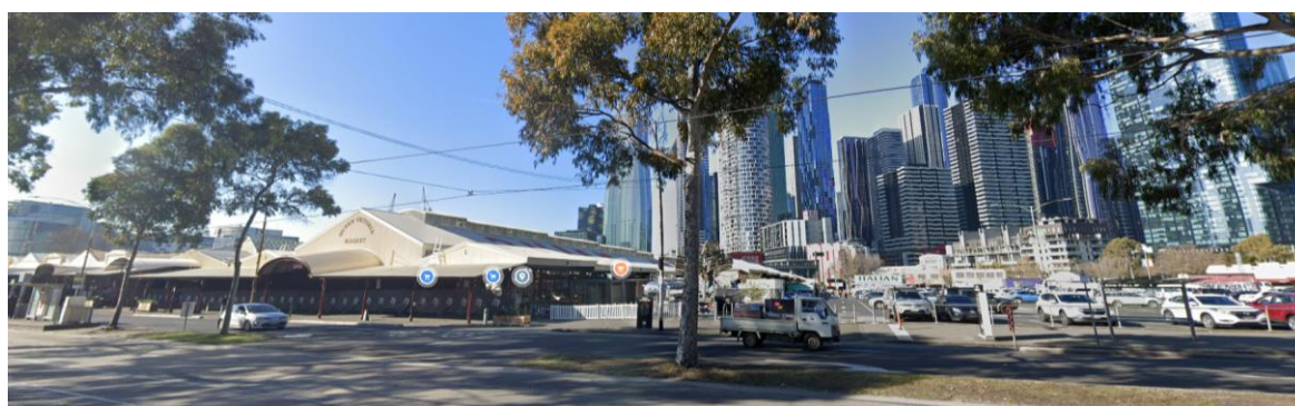
Figure 13. K and L Shed (picture right) in relation to the carpark. Source: Google Street view, 2022.
