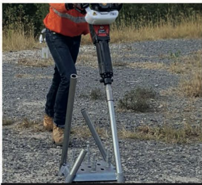
JACK HAMMER MICRO PILES
