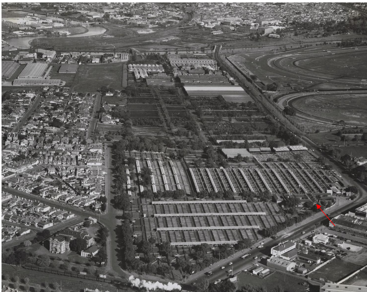
Figure 7. Aerial overview of Kensington c. 1985, with the Maribyrnong River to the south (top), Flemington Racecourse (right) and the Newmarket Saleyards (bottom right, indicated). Source: Pratt, C.D. 1953. Aerial view looking west showing Kensington Stock and Sale Yards. Digitised photograph. The State Library of Victoria (website). Accessed 4 October 2024. http://handle.slv.vic.gov.au/10381/386131
