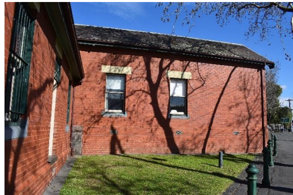
Figure 38. The northern elevation of B1(2) facing Racecourse Road.
