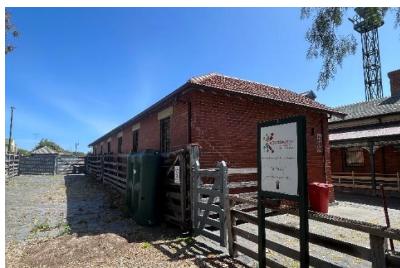
Figure 42. Overview of the northeastern and southeastern elevations.
