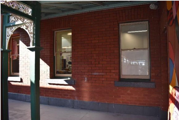
Figure 31. Section of the internal verandah to the C shaped building.
