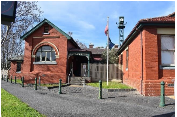
Figure 34. Overview of part of the primary façades facing Racecourse Road.
