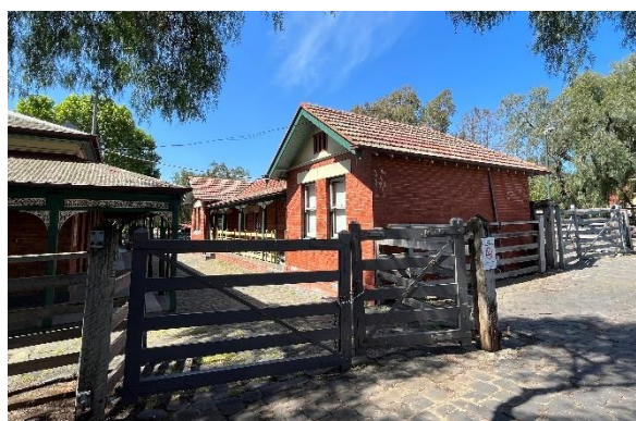
Figure 41. Overview of B2 from Serong Street.
