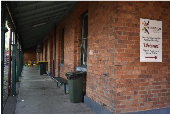
Figure 20. Oblique view of the southwestern elevation.
