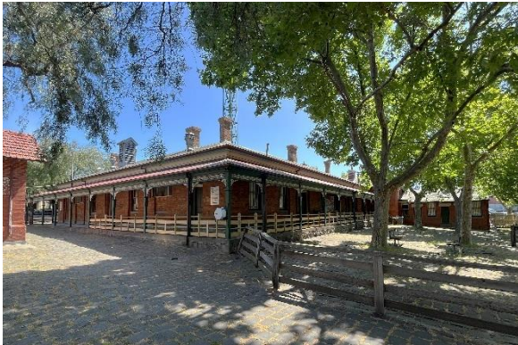
Figure 23. Overview of the northeastern and southeastern elevations, with surrounding bluestone paving.
