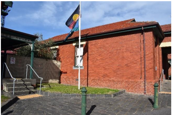
Figure 36. Overview of the northern elevation from the public domain.
