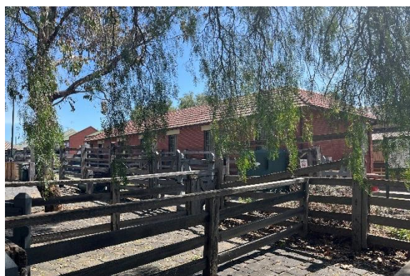
Figure 44. Overview of B2 looking southwest from the remaining stockyard pens.
