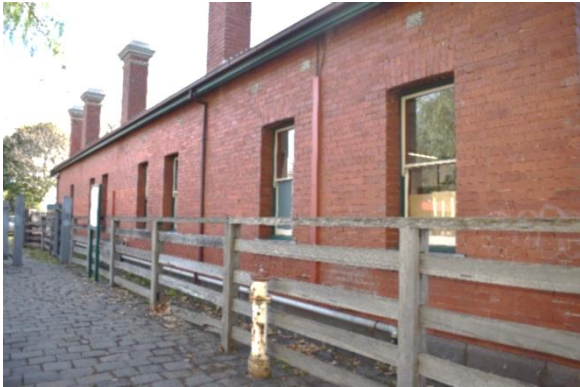
Figure 27. Overview of the southwestern elevation of B1(2).
