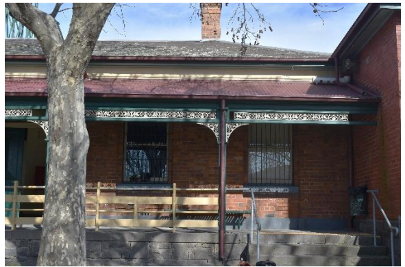
Figure 26. Partial view of the northern most corner of the northeastern elevation.
