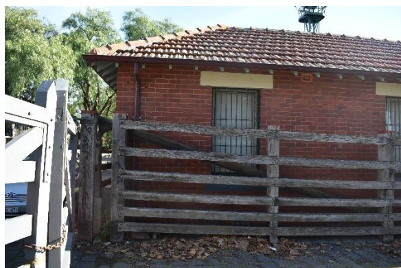
Figure 43. Partial view of the southern end of B2.
