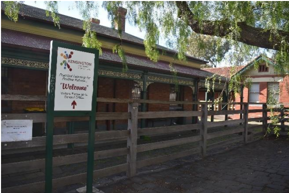
Figure 21. View of the southwestern elevation from Serong Street.
