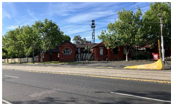
Figure 13. View of the primary façades facing Racecourse Road.
