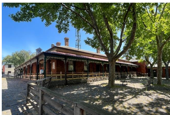
Figure 16. Overview of the northeast and northwestern elevations and bluestone courtyard.
