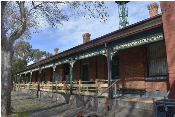
Figure 25. Overview of the northeastern elevation.
