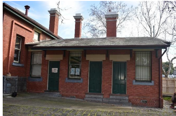
Figure 40. Southeast facing internal elevation.
