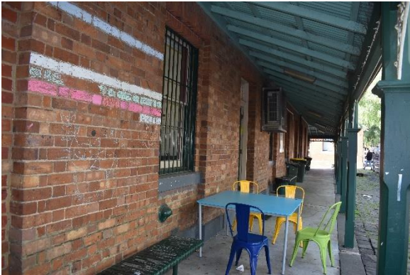
Figure 19. Oblique of the southwestern elevation, looking east
