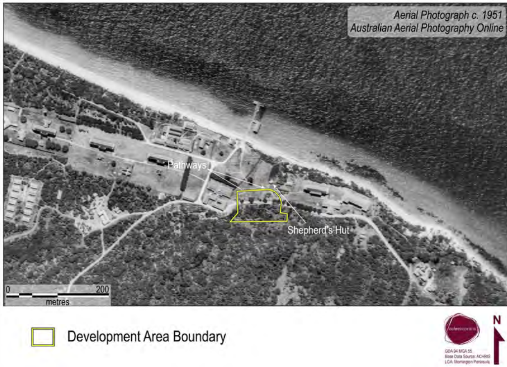
Figure 29 – Aerial photograph of the development area c. 1951. Image source: AAPO.
