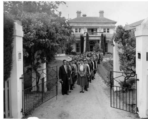
Figure 6: View of the house at the time of its occupation by the Melbourne Bible Institute (c.1950s) showing interwar style piers and gate, in-go entry with piered gateway and timber picket fence. Source: Melbourne Bible Institute Archive.
