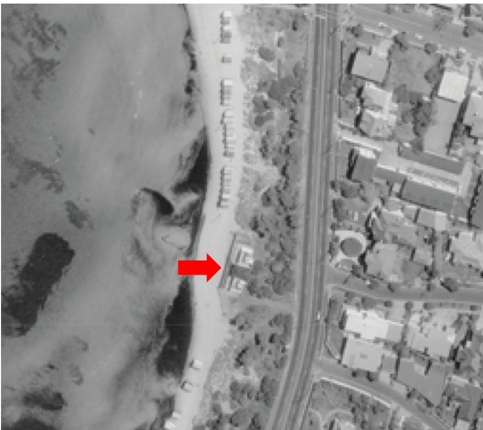
Figure 11 Aerial photograph showing location of kiosk building indicated, 1977 Source: Historical Aerial Photography Collection, Landata, Secure Electronic Registries Victoria
