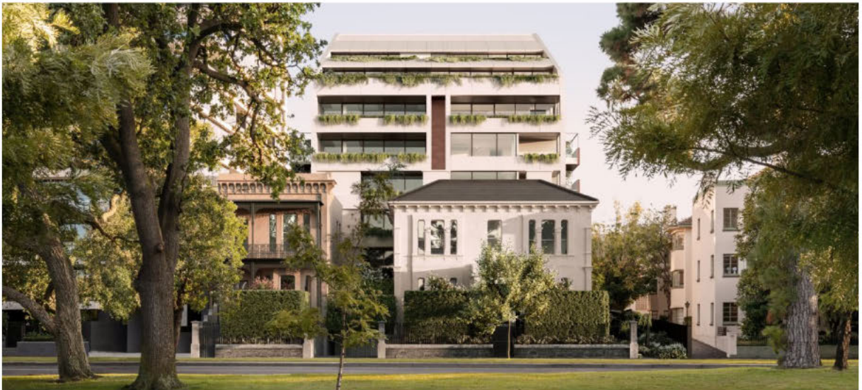
Figure 2 – Render showing the proposed new envelope behind the Victorian buildings at 250 and 260 Clarendon Street to the west of the site.
