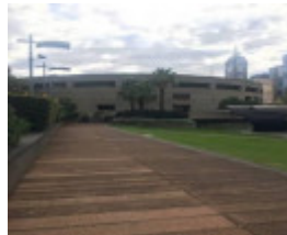
2019_Walkway rear of Forward Surge.jpg
