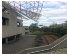
2019_Rear of Theatres Building.jpg
