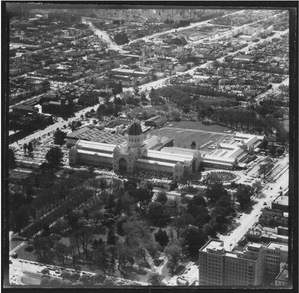
Figure 67: Payens, Jim. (1962) Photograph - Aerial View of the Royal Exhibition Building, Carlton, Victoria, Apr 1962. MM 134769. Museums Victoria Collection. Melbourne, Australia.
