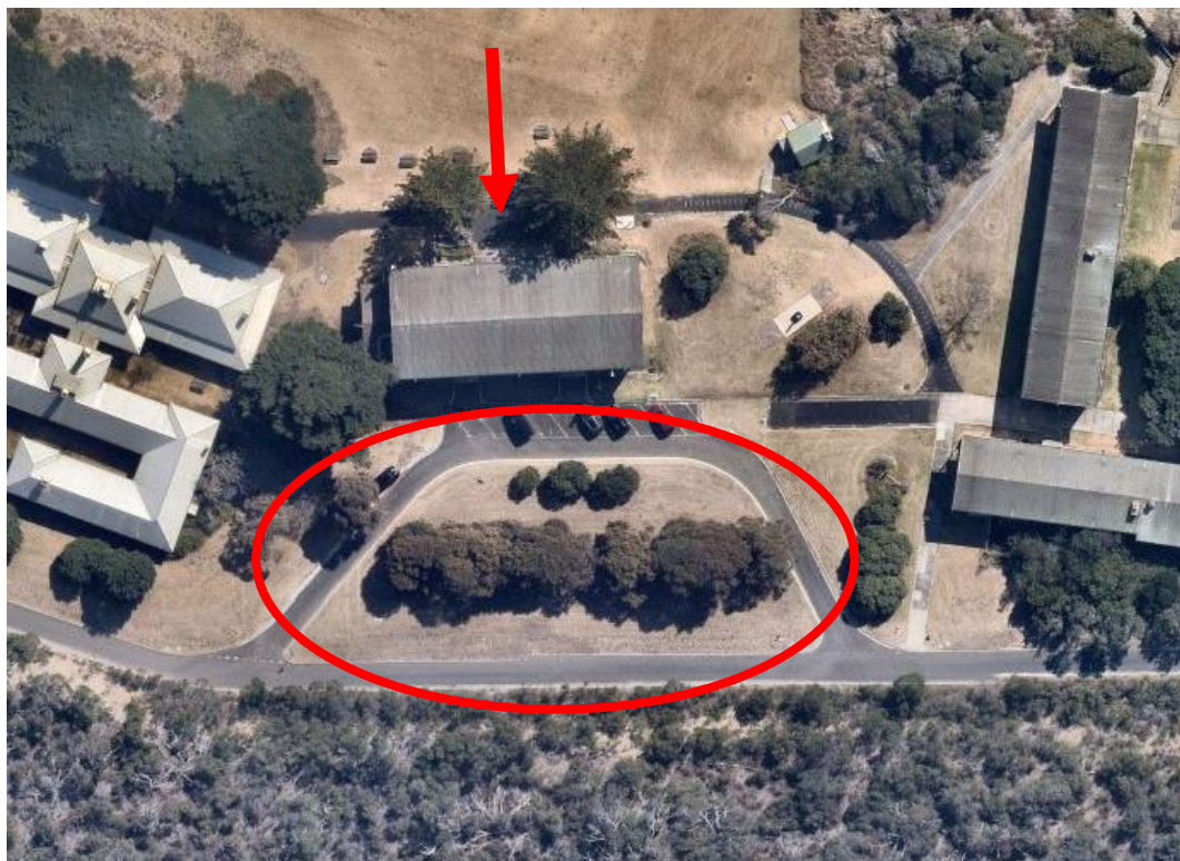
Figure 8 Detail of the above image approximately indicating the location of the proposed building with Badcoe Hall to the north (indicated by the red arrow); north is at the top of the image Source: Nearmap, image date March 2024
