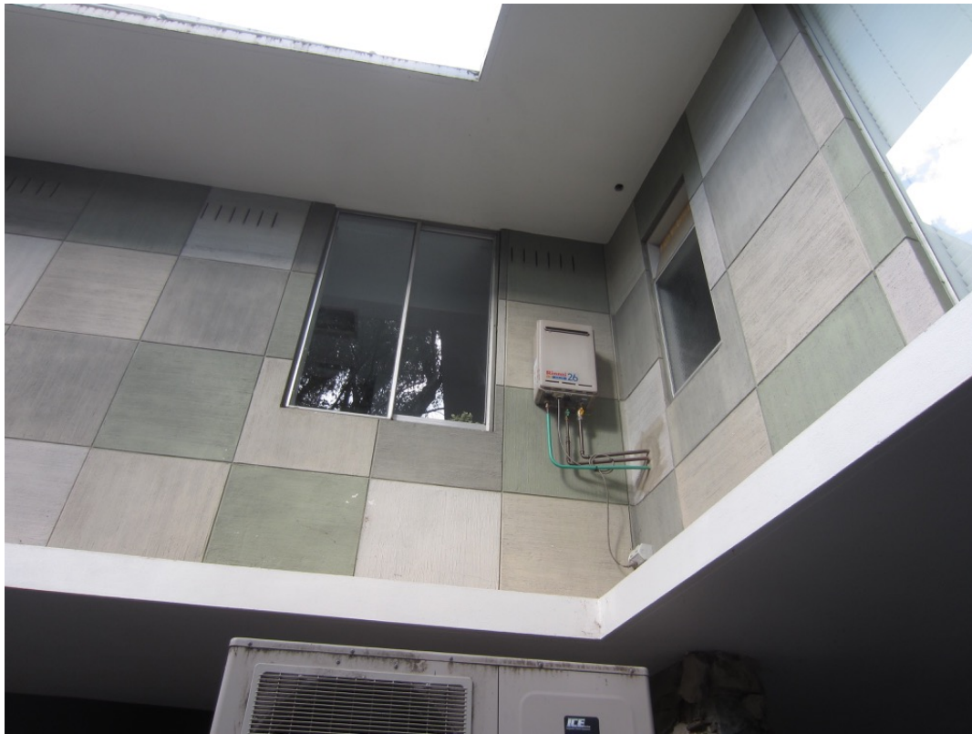
Figure 14 The first floor rear wall showing the coloured square rendered cladding.
