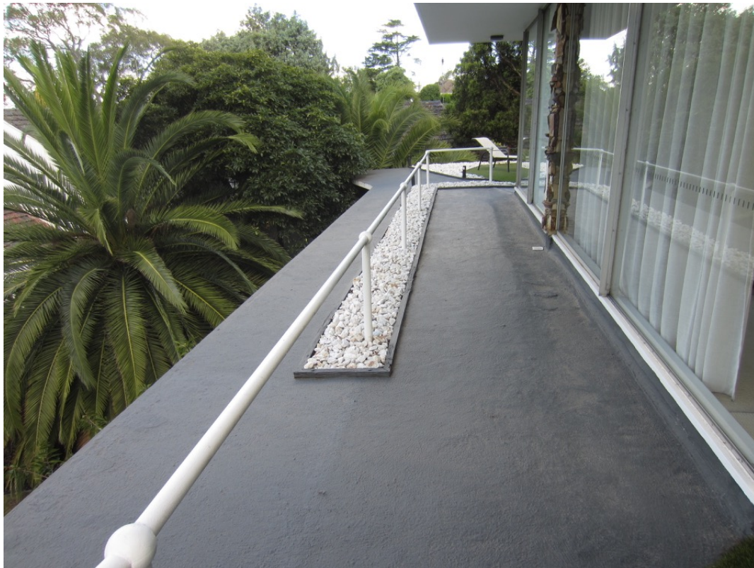
Figure 18 Second storey roof deck with steel rail added in 1992.
