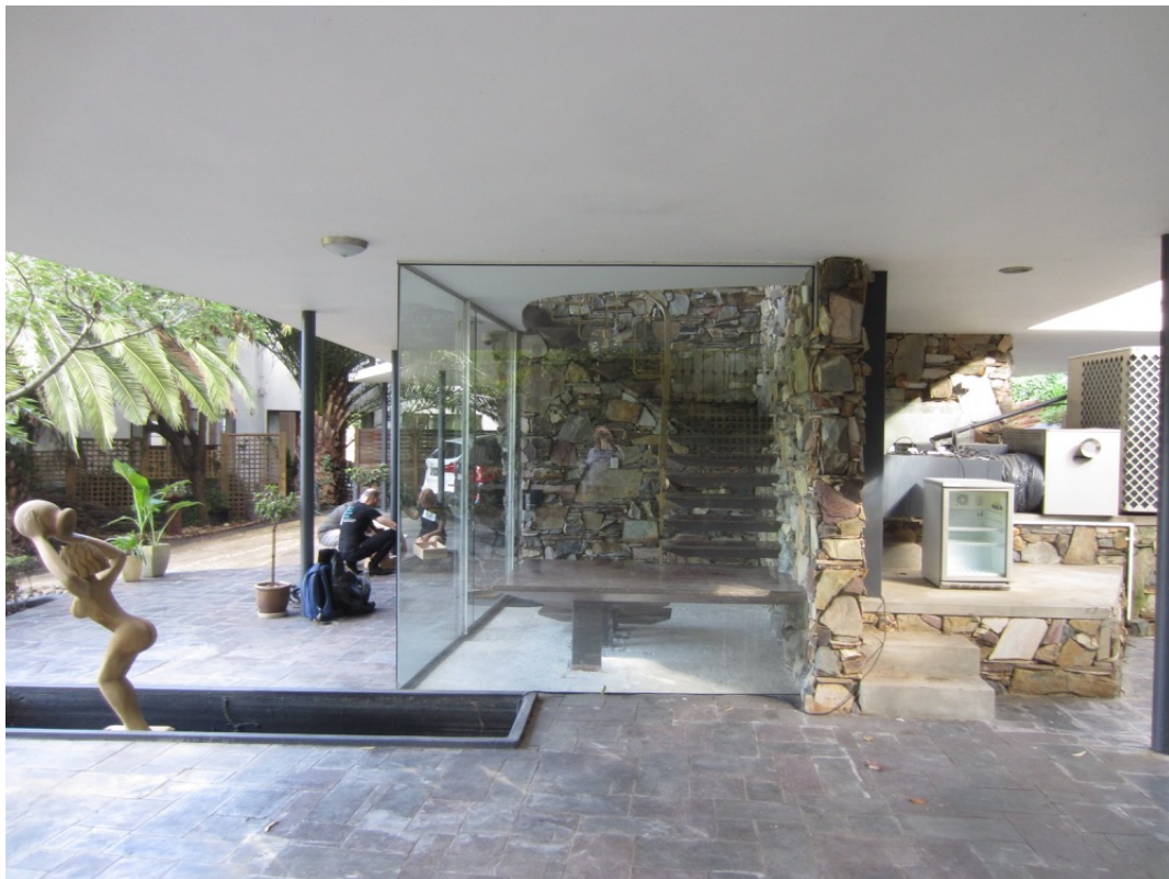
Figure 11 The entrance undercroft from the west showing the simple glass box surrounding the staircase.
