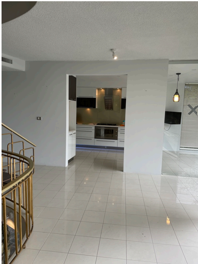
Figure 26 View from the staircase towards the kitchen showing the sections of wall planned to be removed.
