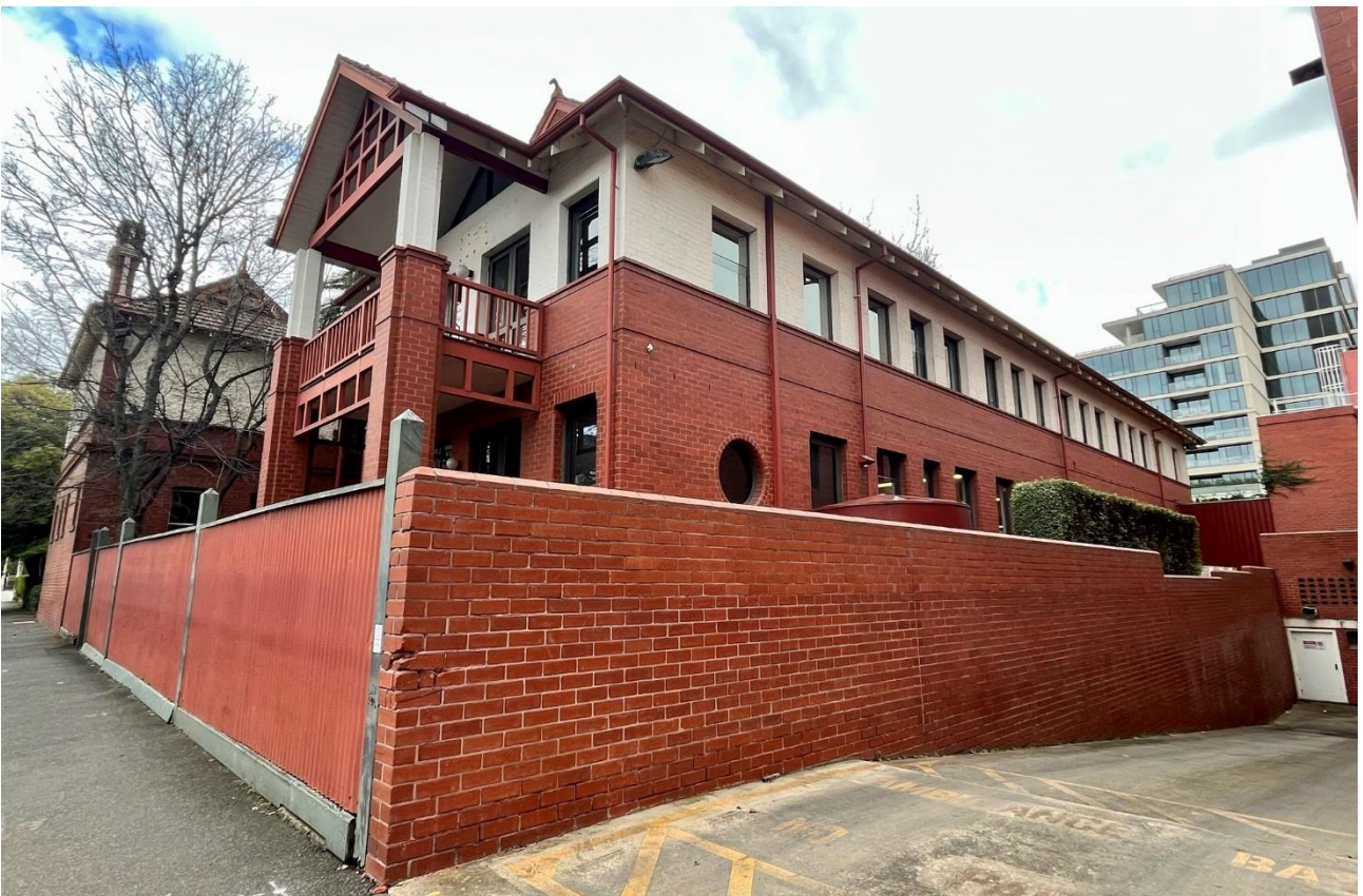
Figure 3 – 1982 addition viewed from the north
