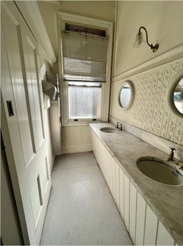
Figure 4 – The existing first floor bathroom looking west.
