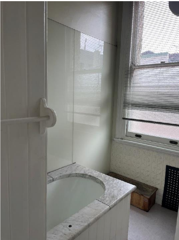
Figure 5 – The bathtub to the first floor bathroom.
