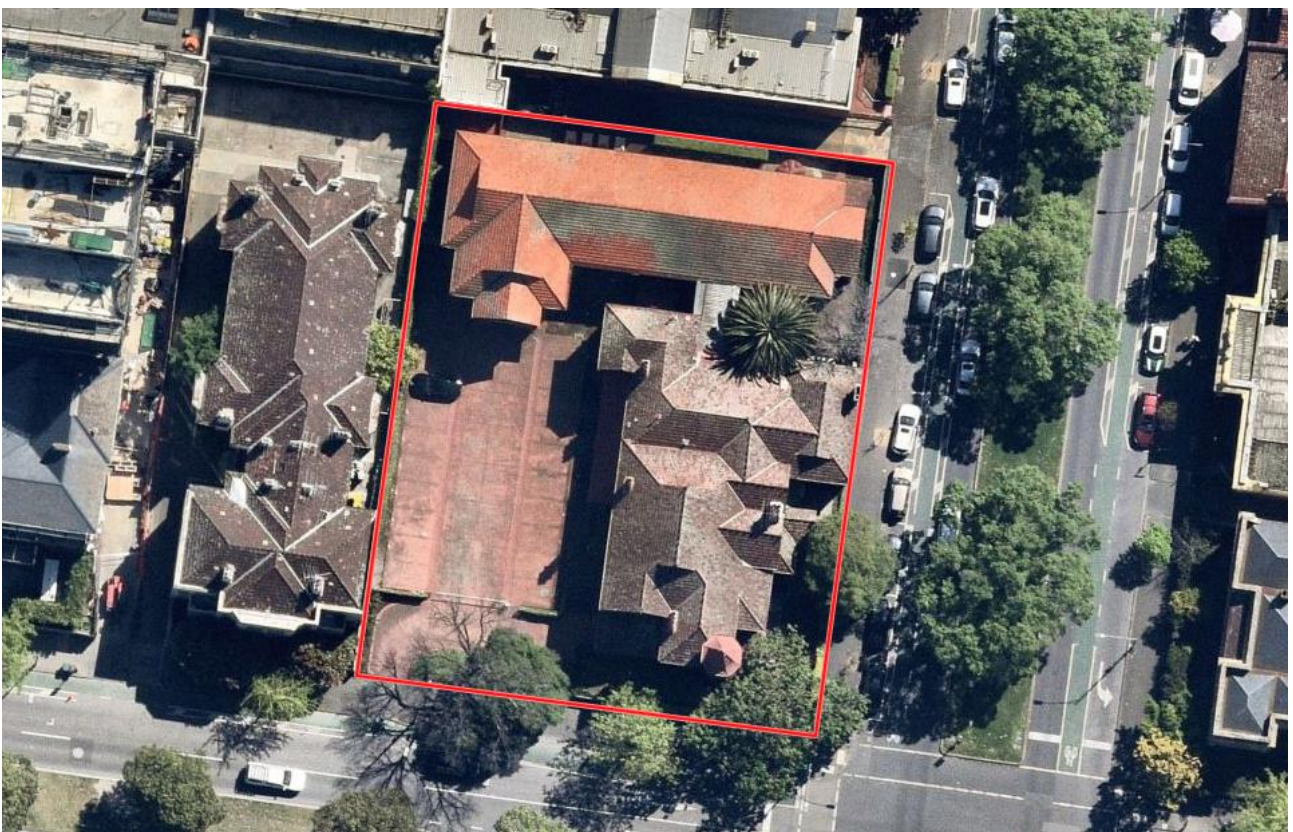
Figure 1 - Aerial photograph showing the location of the subject site at 1-19 Clarendon Street, East Melbourne, outlined in red
