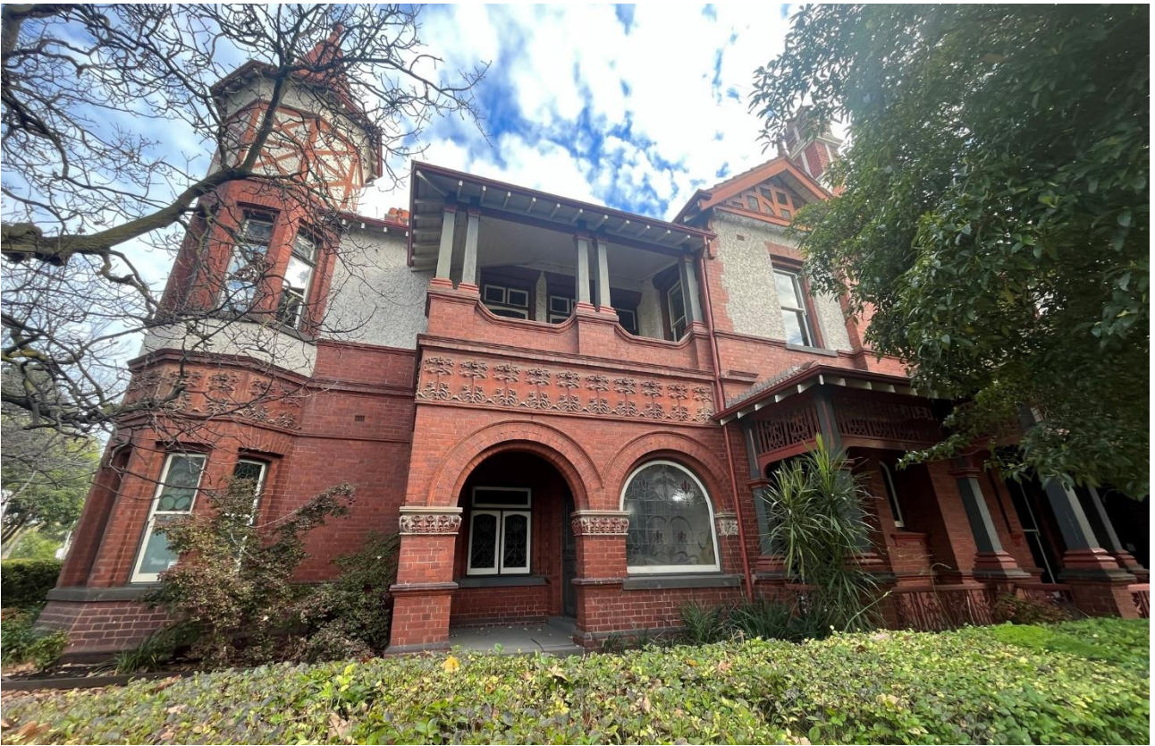
Figure 2 – Corner tower and ground floor entrance portico of St Hilda's House
