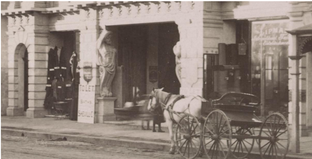
Figure 6: Detail of Chapel Street facade.-Note the recessed central vestibule with rusticated entry reveals and flanking caryatids. (Source: SLV, H39357, 232)
