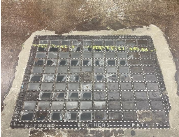
Figure 27: Prismatic floor light, central arcade ground floor level.
