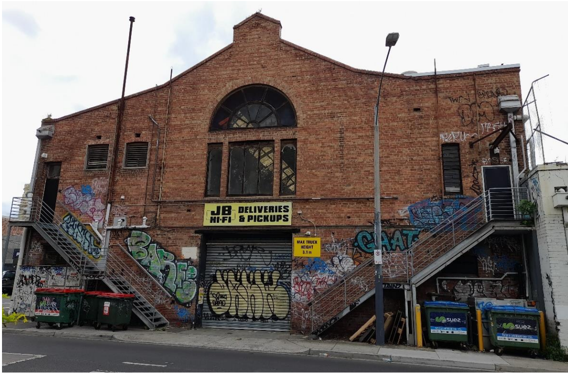
Figure 14: Prahran Arcade from Little Chapel Street.
