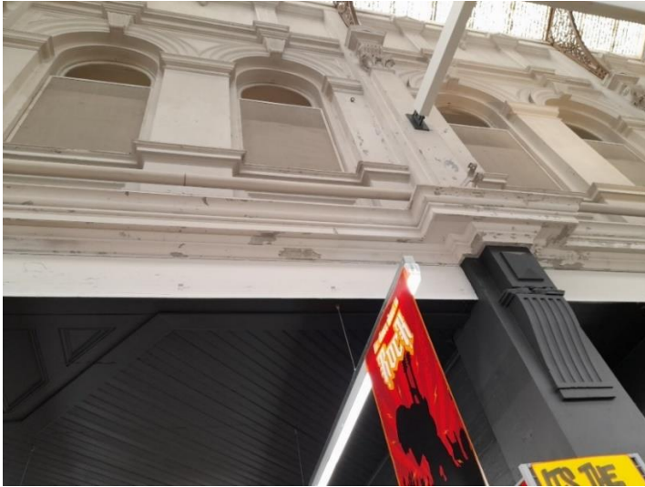
Figure 21: Upper arcade walls.
