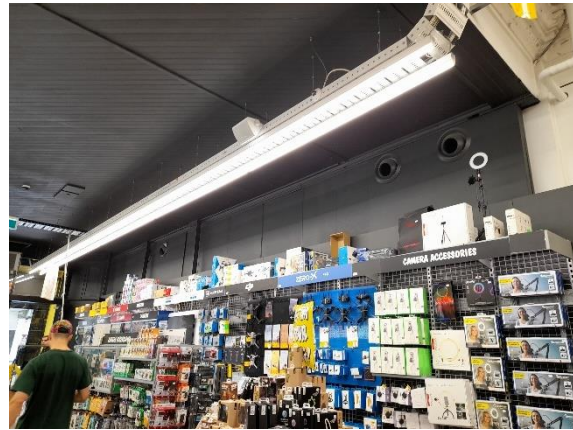
Figure 30: Cable trays, ducts installed within highlights
