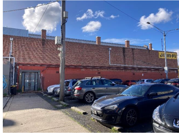
Figure 16: South (side) elevation facing Council carpark.
