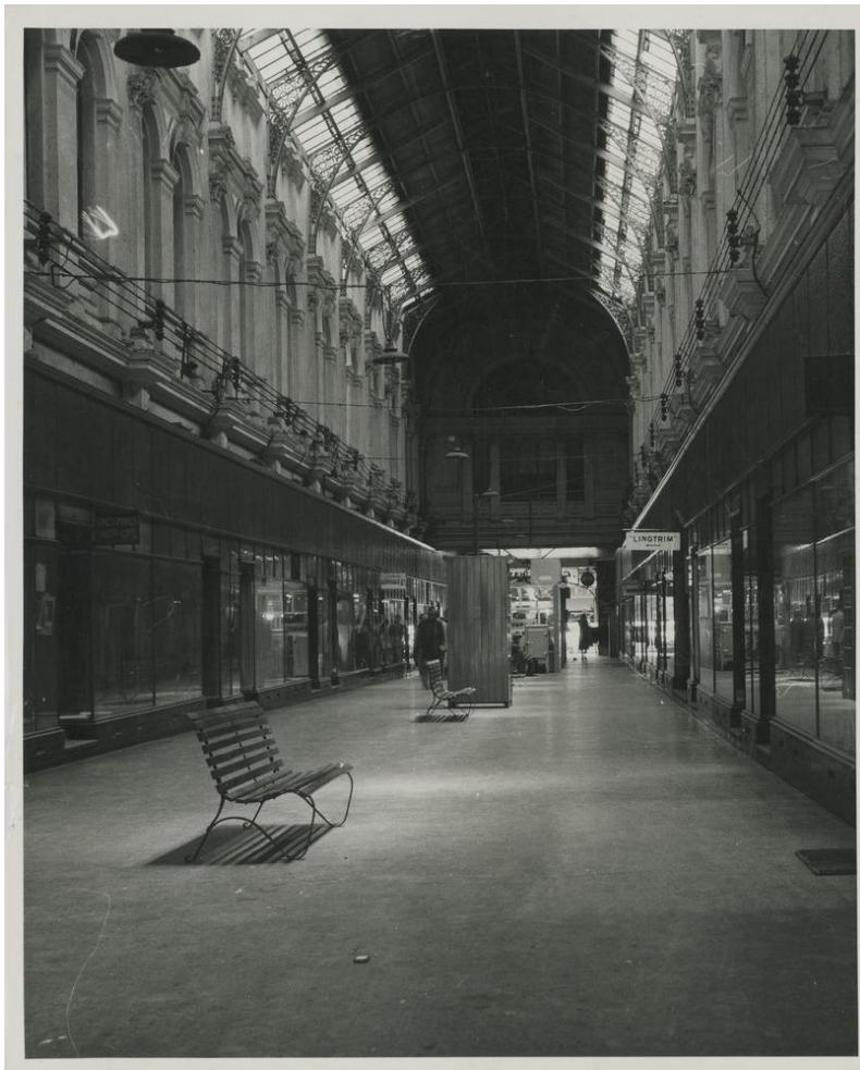
Figure 10: Circa 1920s, Prahran Arcade, Chapel Street Prahran VIC (Source: SLV, H2009, 154 10)
