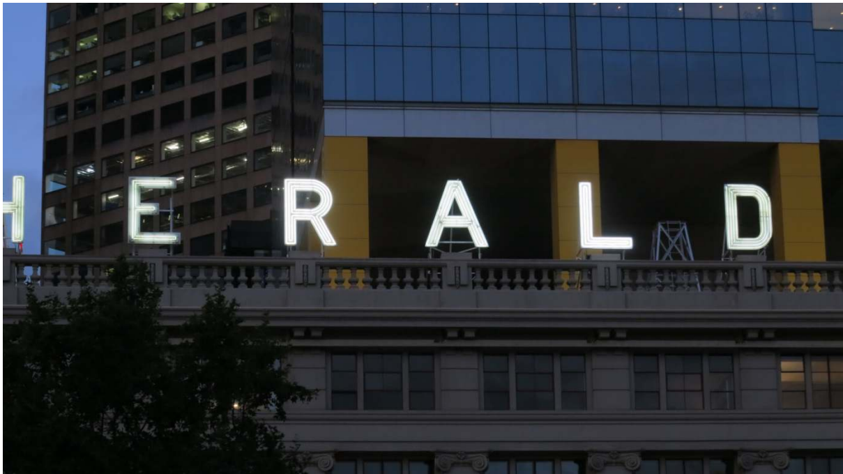
Existing Neon gas letters: H, E,& D (E not fully functioning)
