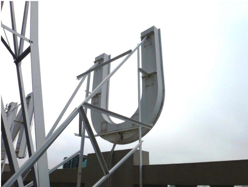
Rear side of letter and support structure in steel. What can be seen in this illustration will all remain
