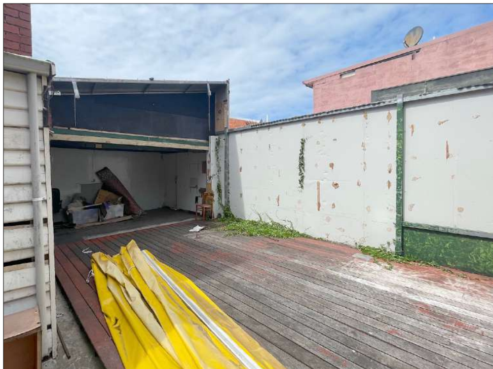
Figure 11 The yard at the south-east corner of the site.
