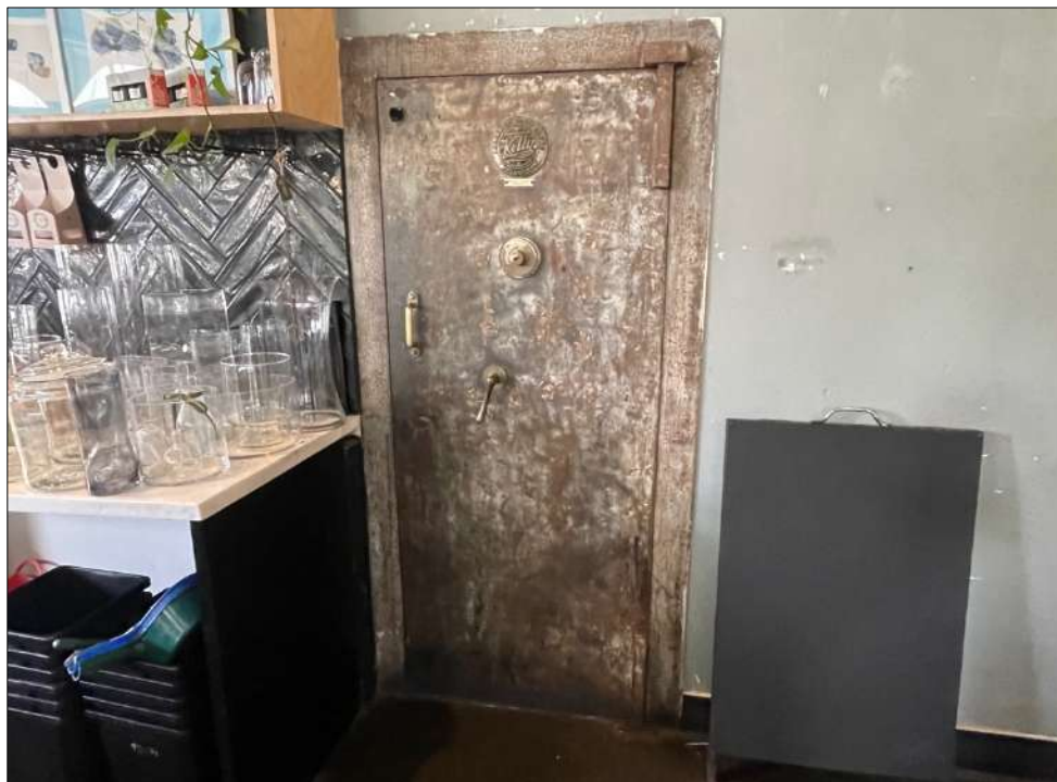
Figure 15 The bank vault door.
