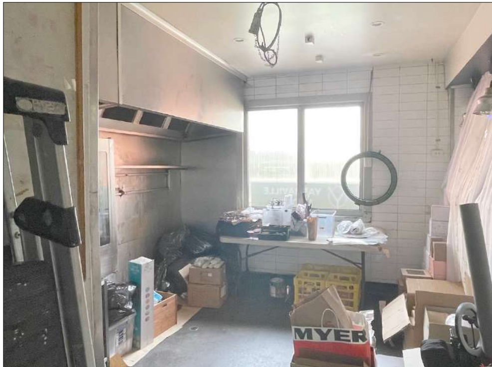
Figure 16 The commercial kitchen, occupying the single-storey post war addition to the south side of the banking chamber.
