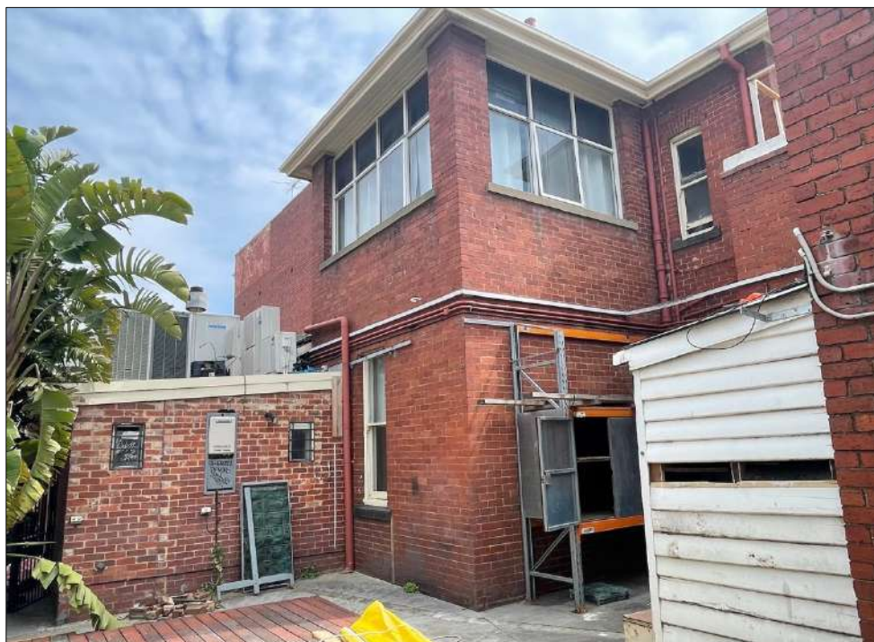
Figure 9 Partial view of the south elevation looking north-west.
