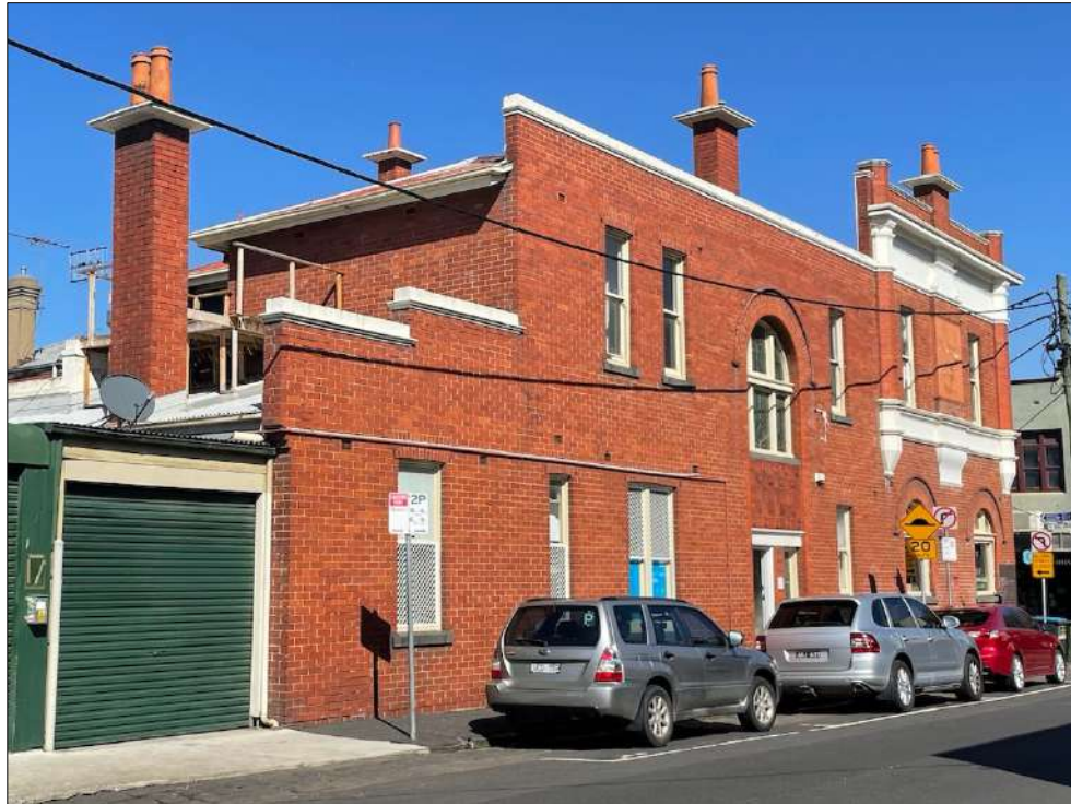
Figure 8 The Canterbury Street (north) elevation.
