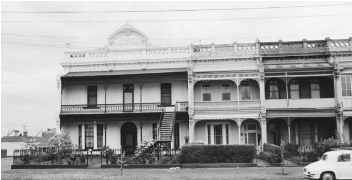
Hambleton House (left) and terraces. (Source: Committee for Urban Action, 1970-1974, SLV: CUAMSM251/1, Image 2)
