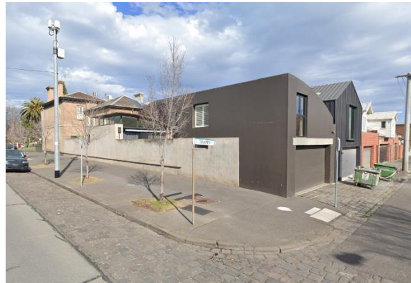
46 and 48 St Vincent Place North – rear additions (Source: Nearmap, August 2022)
