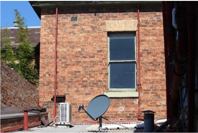
Rear window with cream brick lintel
