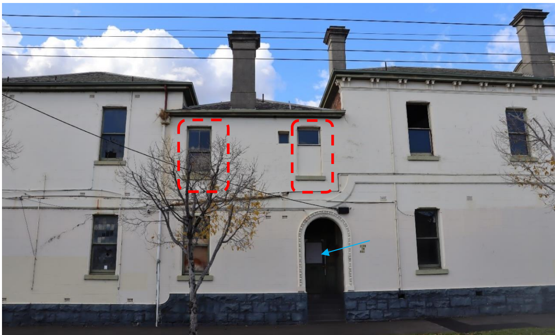
Montague Street elevation - rear service wing (1877). The highlighted windows (dashed red) would become partial blind niches. The non-original side entry door (blue arrow) would be replaced.
