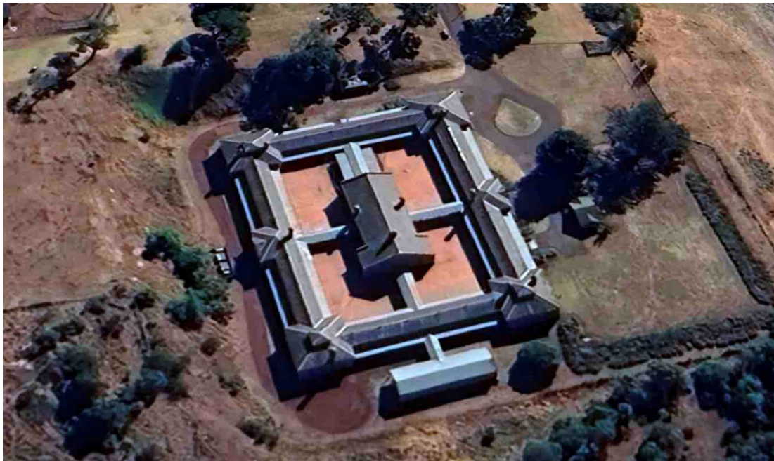
Figure 1 Aerial of the former Female Refractory Ward (B25) with the flat airing court with the Privy (B19) to the east.
