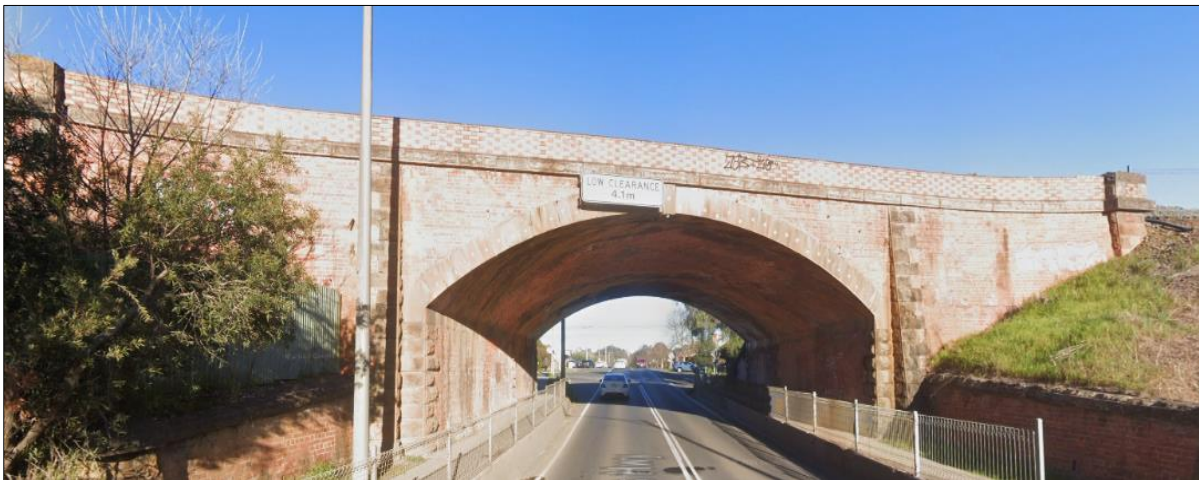
Midland Hwy Bridge, Castlemaine 2024 (Google Maps).
