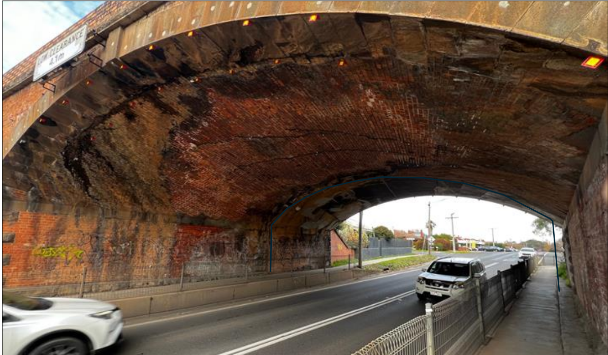
Fig. 7. Midland Hwy Bridge Soffit (2024)
