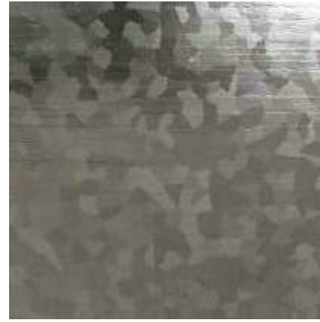
FACADE / ROOF STEEL FRAMEWORK HOT-DIPPED GALVANISED
