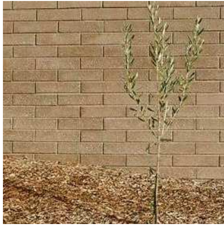
MASONARY BRICKS ADBRI MASONARY OR SIMILAR LIGHT SANDY TONES 230MM X 110MM X 76MM
