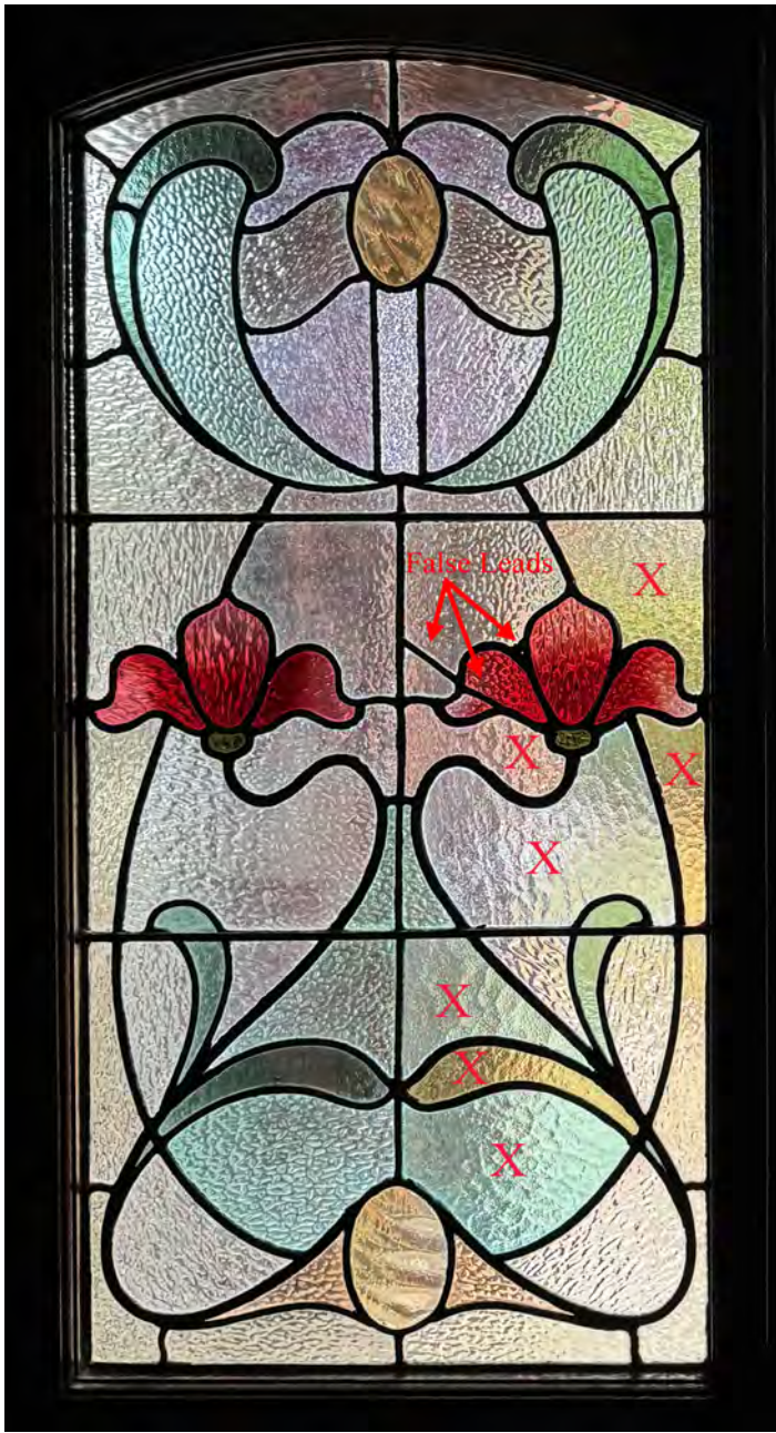
WG.03 - LHS Multiple glass replacements and addition of false leads over cracked pieces of glass.
