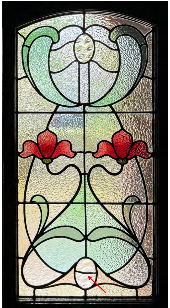
WG.03 - False lead over a crack in a piece of Venetian glass.
