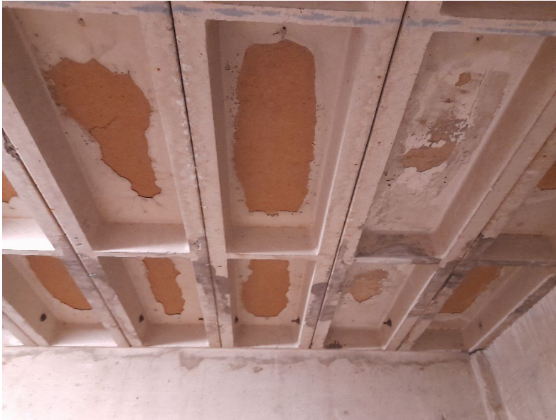
◀ Wilson Hall, basement. Underside of waffle slab.
