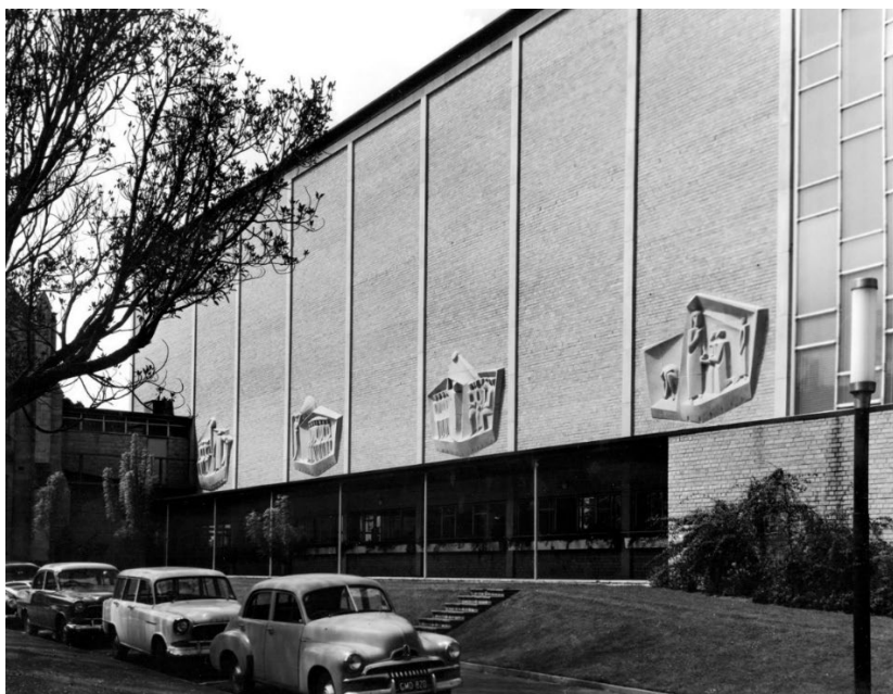
◀ Wilson Hall, west elevation. Note the delineation between the recessive character of the covered way below and the elevated sculptural wall above the canopy. Photograph by Wolfgang Sievers, 1959 (Source: State Library Victoria)
