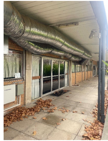
Top: View through Cenotaph Lawn from South Lawn to west elevation of Wilson Hall. Bottom Covered way (L-R): Screened AHU; External flexible duct and plenum connection box; View south.
