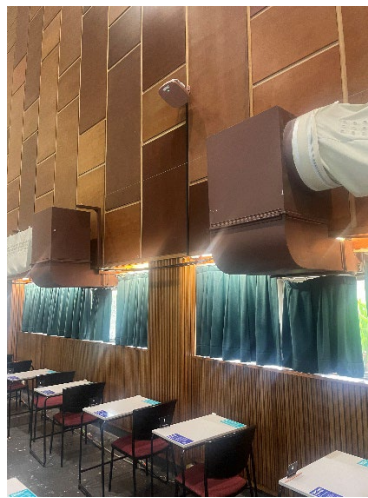
Existing internal fabric ductwork and internal plenum connection boxes
