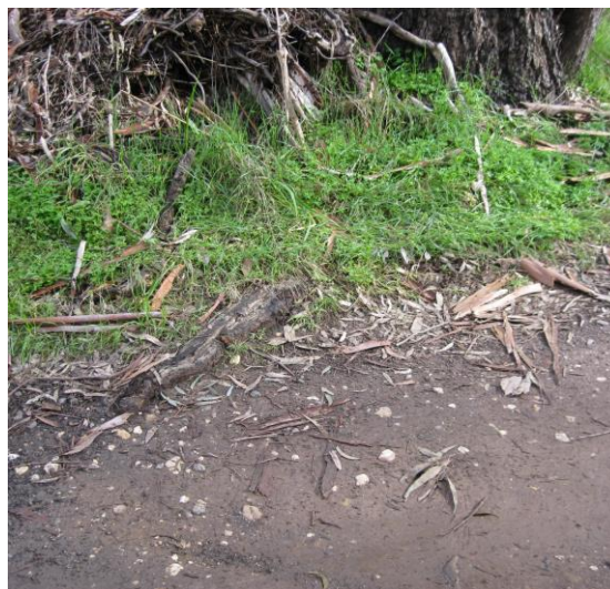
Figure 4. Large structural roots located under the existing roadway
