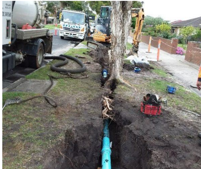
Figure 11. Hydro excavation used to sensitively install utility pipes. (Hydrox Root Controllers).
