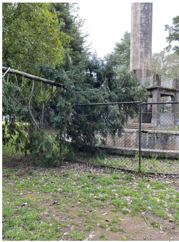
Overhanging tree branch to be removed
