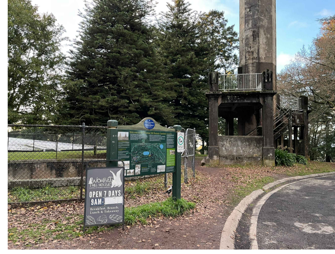
6 Existing signage in front of Day Basin 22.08.2022
