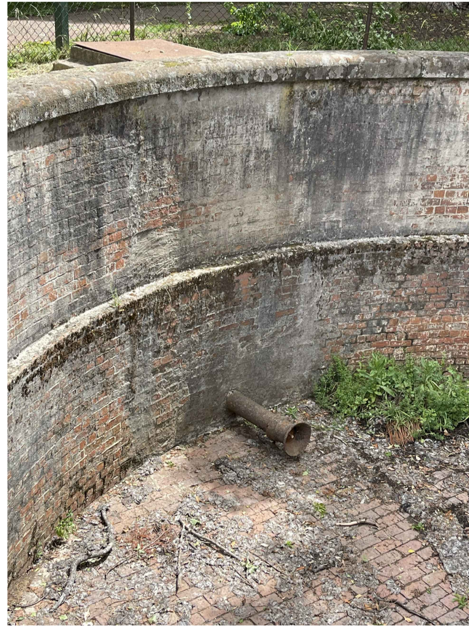
9 View into Day Basin showing cast iron pipework 30.11.2023
