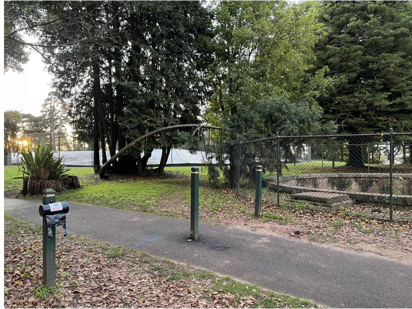
1 View from asphalt path to covered reservoir, showing overhanging branch 22.08.2022
