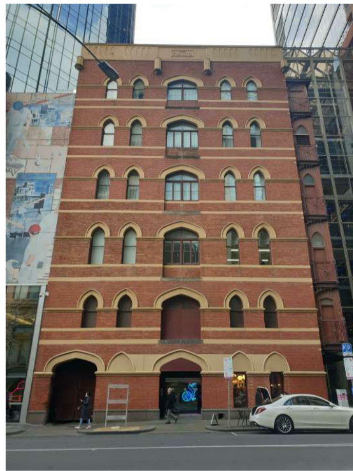
Rear elevation of the Rialto building.
