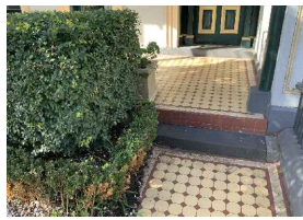
EXISTING FRONT VERANDA TILES TO BE REPLACED
