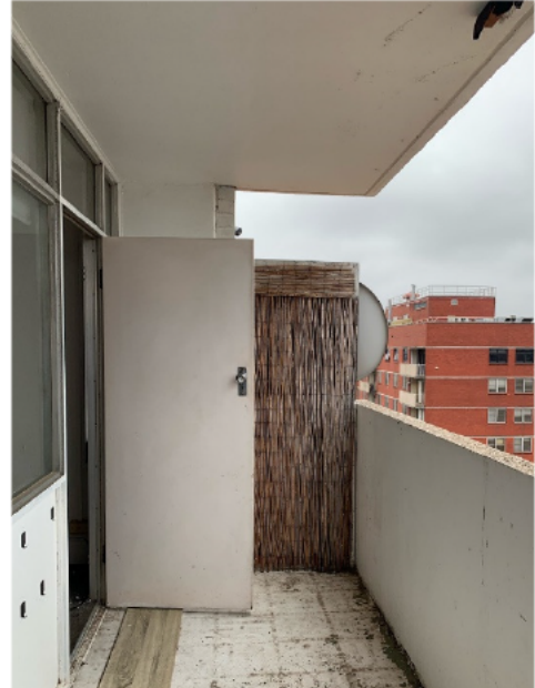
January 2022, View from balcony of an Elgin Street Tower flat towards the Nicholson Street Tower. Source: Homes Victoria.
