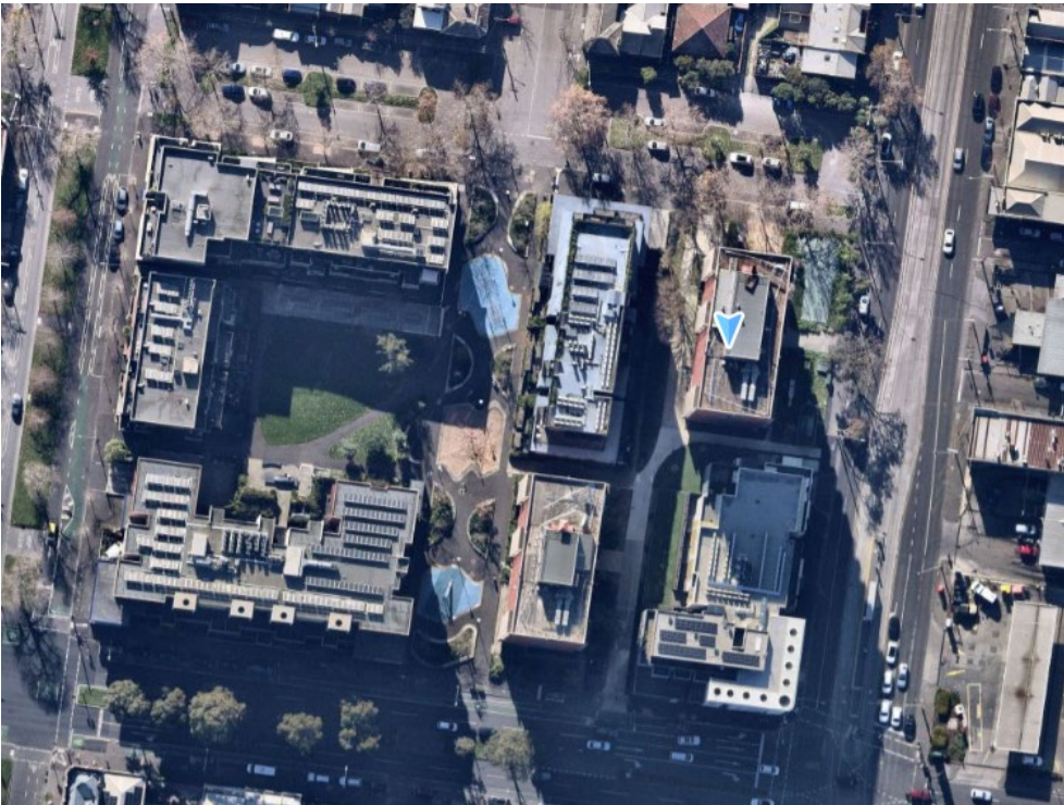
Figure 10 Recent satellite imagery showing the extent of redevelopment across the site Source: Nearmap, capture date 23 June 2024
