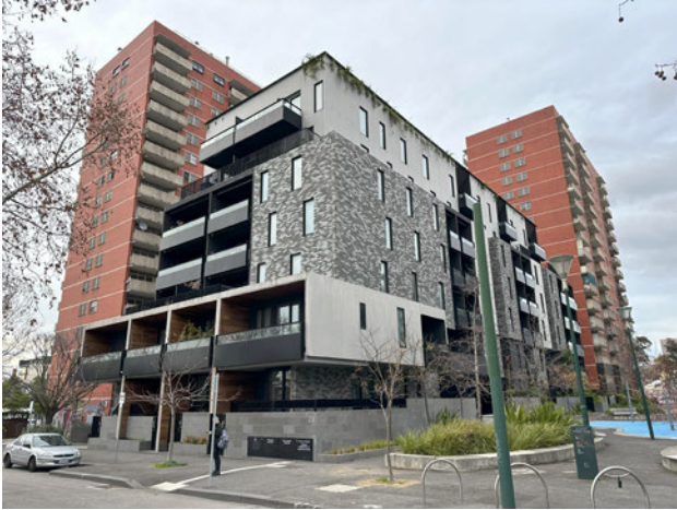
Figure 1 View at the corner of Palmerston Street looking south-east (Lovell Chen, July 2024)
