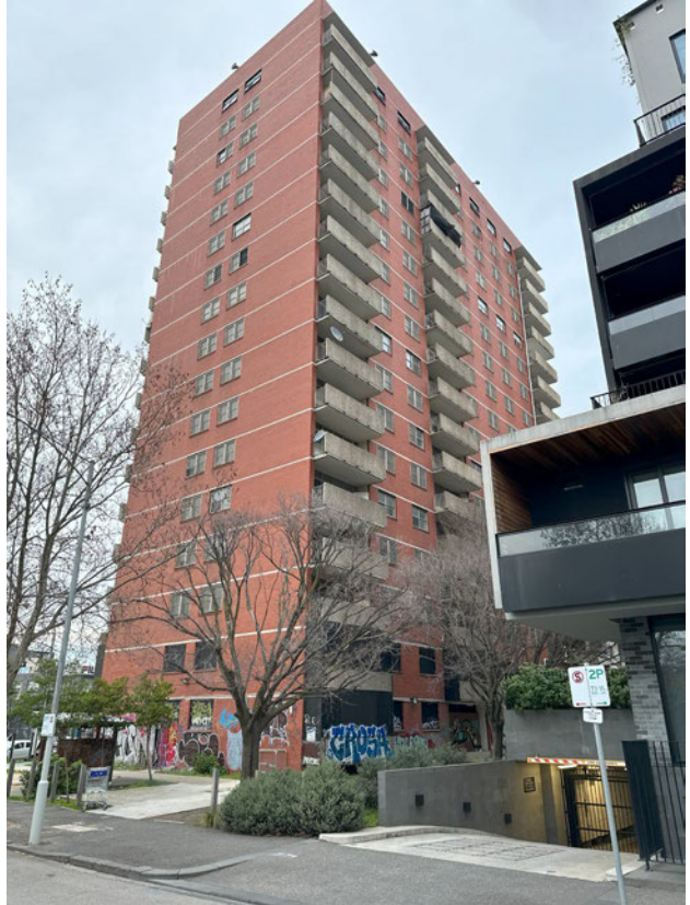
Figure 2 No. 141 Nicholson Street viewed from the north-west (Lovell Chen, July)
