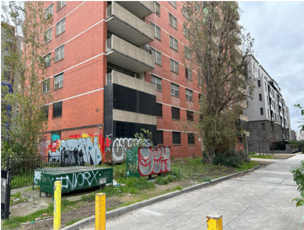
Figure 3 No. 20 Elgin Street, view from the south (Lovell Chen, July 2024)
