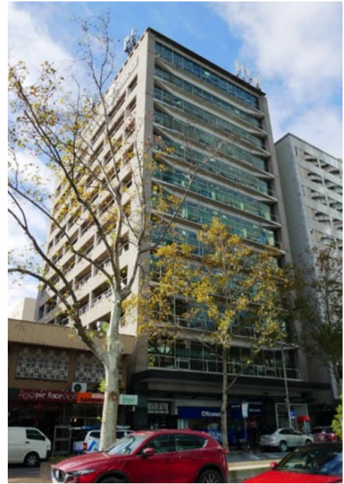
Figure 12 Former Australia Pacific House, 136-144 Exhibition Street, 1975-1978 Source: Statement of Significance, Melbourne Planning Scheme
