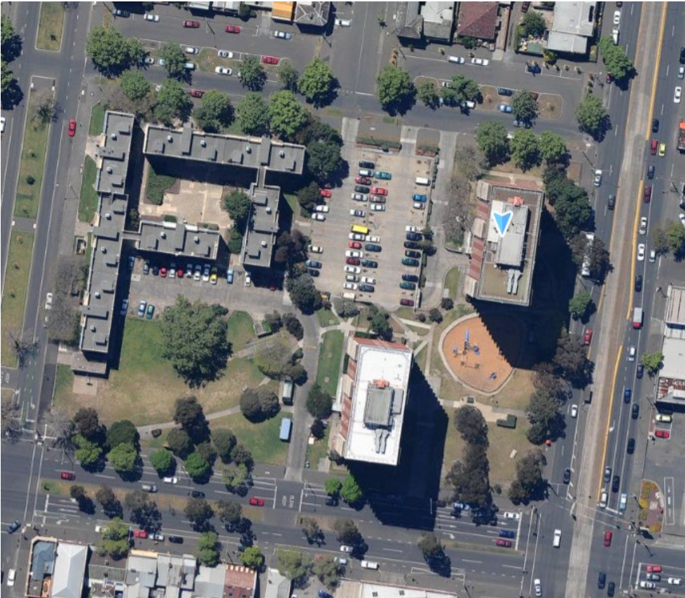
Figure 9 Satellite imagery from 2009 Source: Nearmap, capture date 12 October 2009
