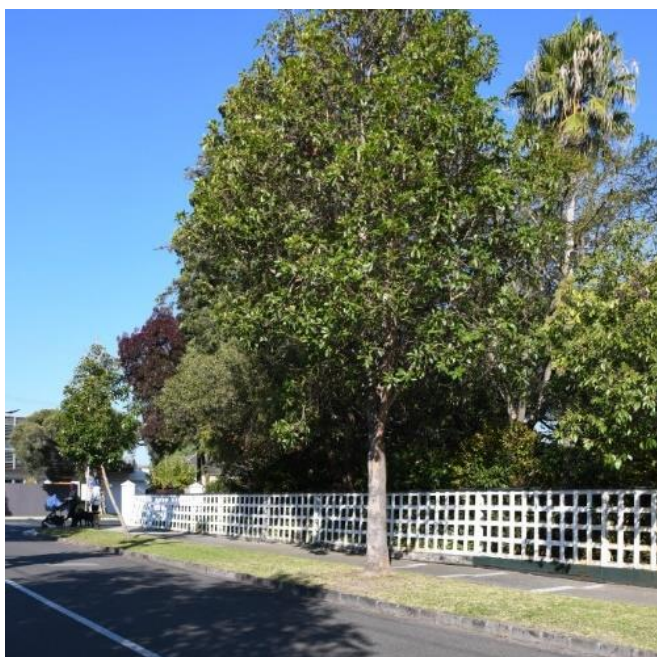
Figure 13 The fence along Halstead Street which will have pedestrian and vehicle gates inserted in it, necessitating the removal of the eucalypt. The fence will otherwise be repaired.
