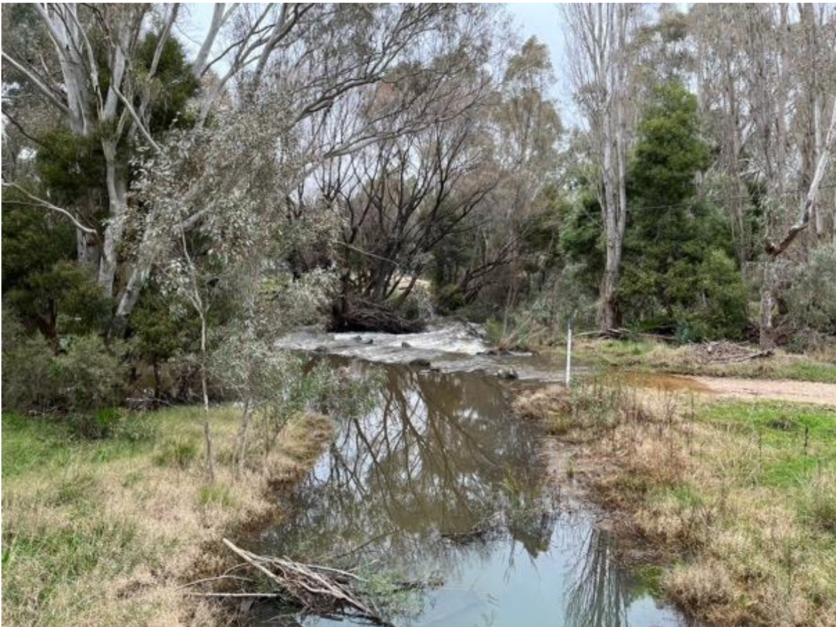
Figure 2-4: Existing crossing, West Facing
