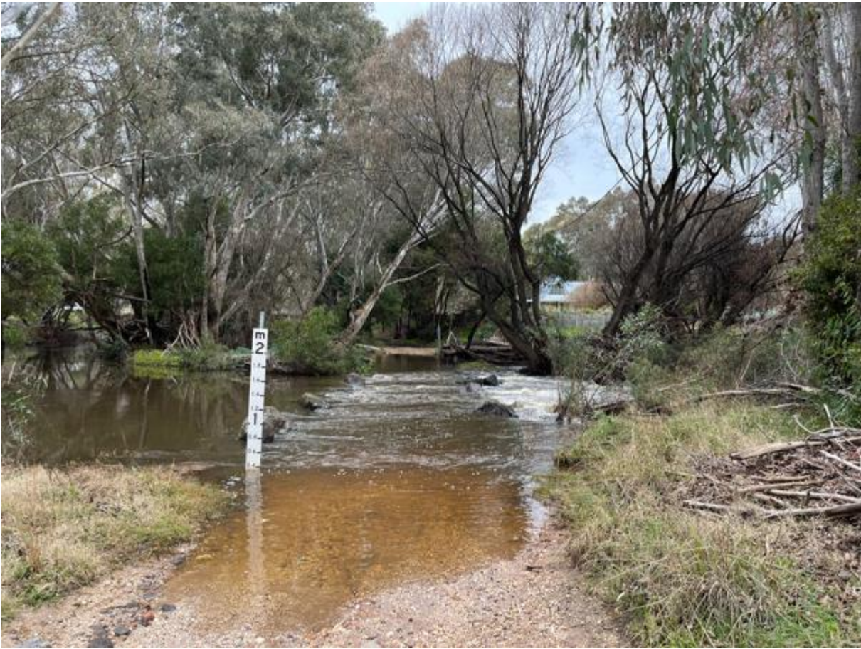
Figure 2-5: Existing crossing, South Facing
