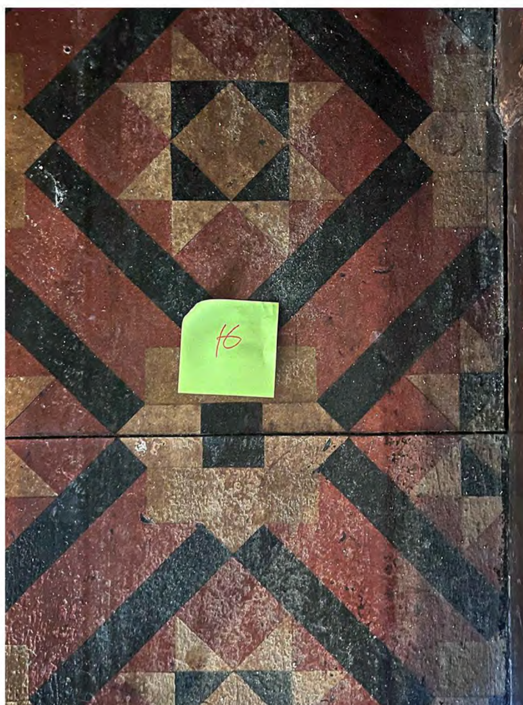
CODE: 1 CONDITION RATING: GOOD NUMBER: 16 GRID LOCATION: 4-DD
