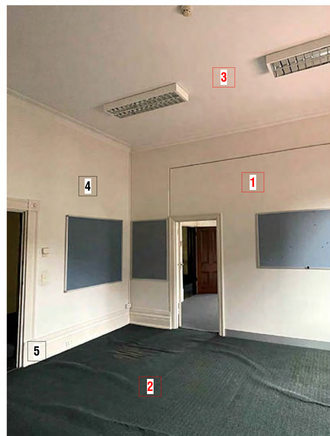
PHOTO - CURRENT VIEW TOWARD NON-ORIGINAL WALL INFILL / OPENING
