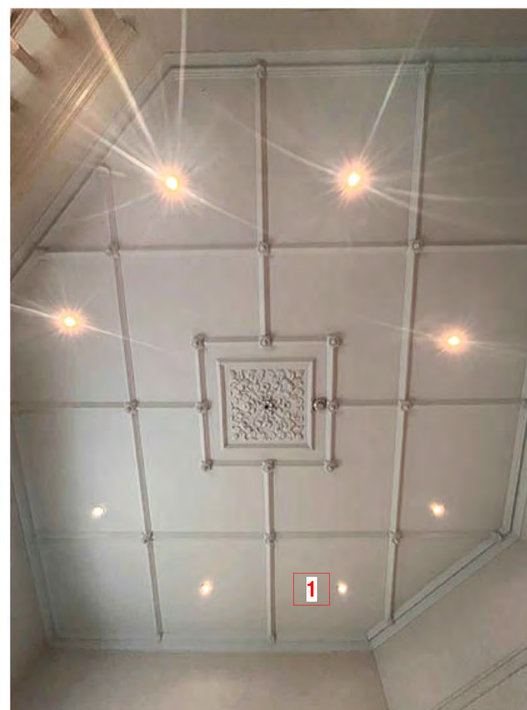
PHOTO - CURRENT VIEW OF CEILING
