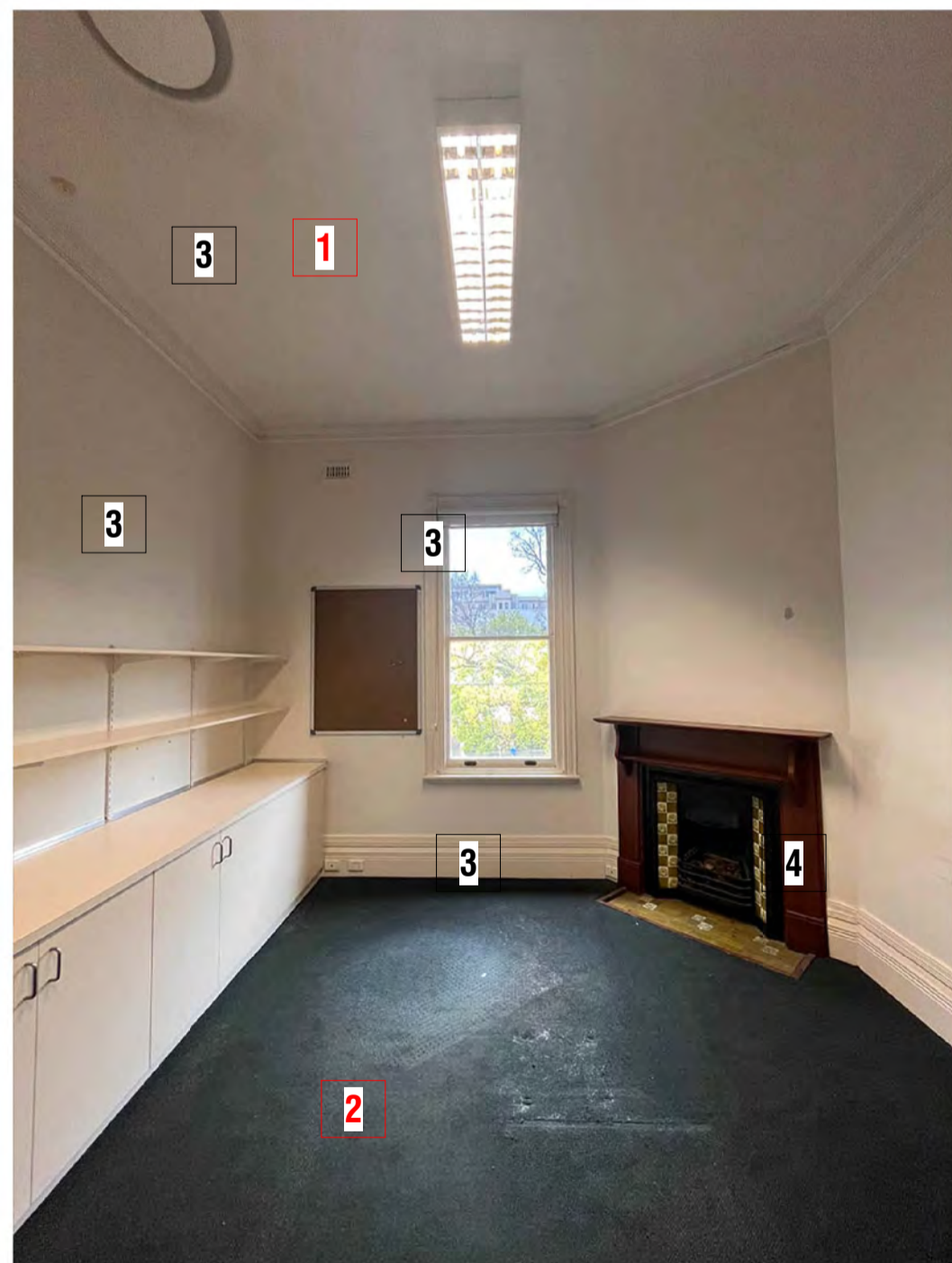
PHOTO - CURRENT VIEW OF ADMINISTRATION ROOM
