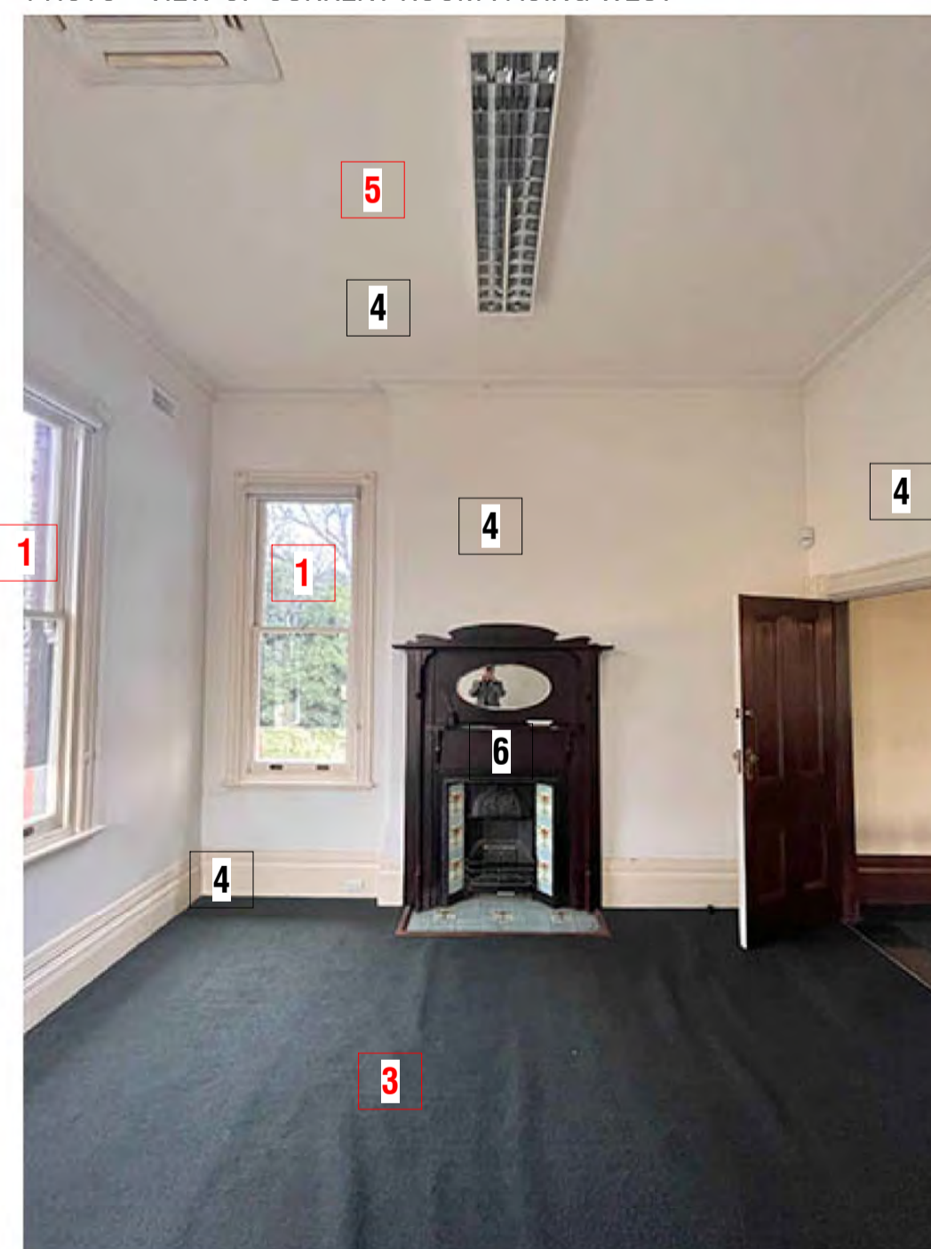
PHOTO - VIEW OF CURRENT ROOM FACING WEST
