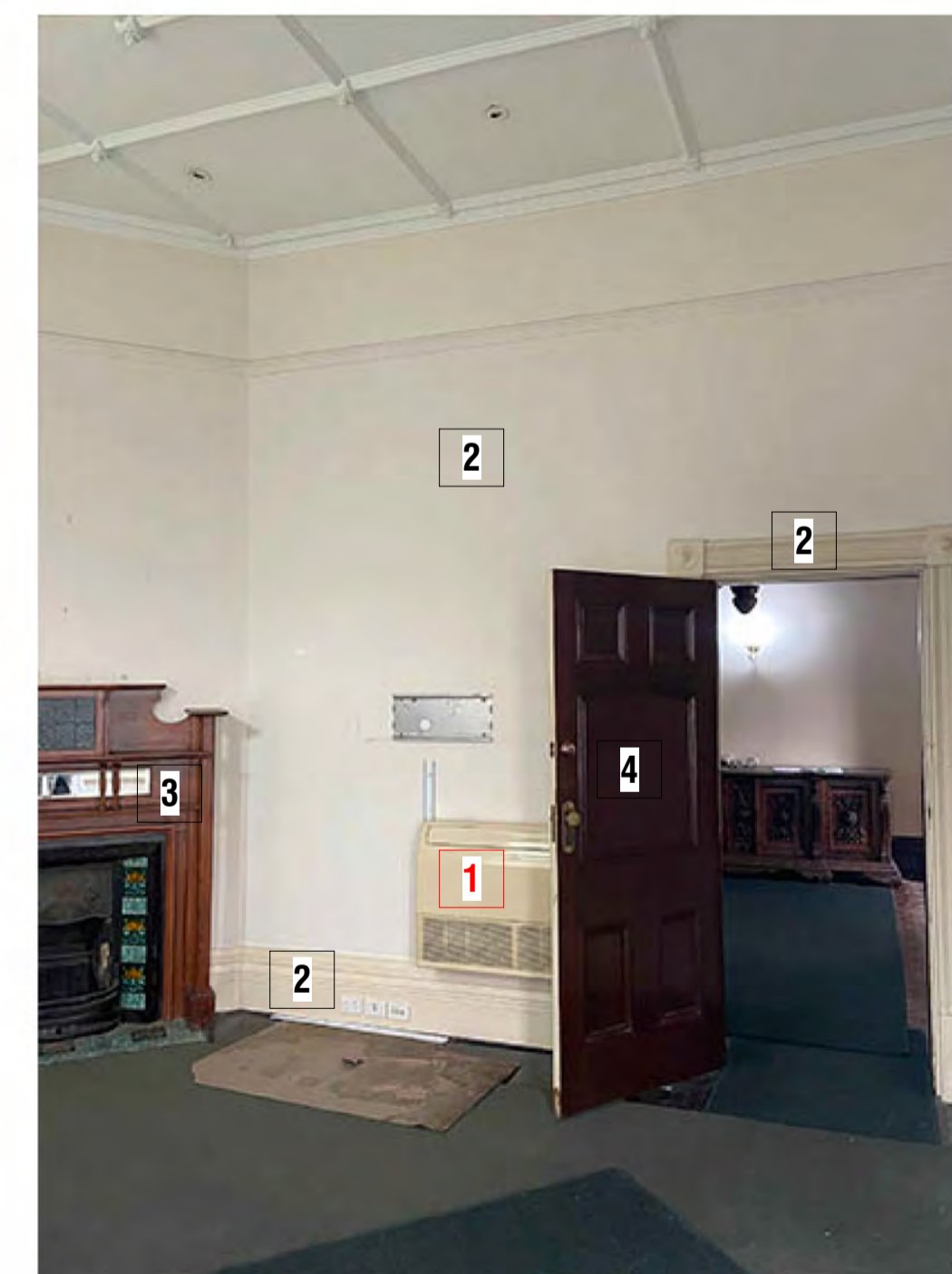
PHOTO - CURRENT VIEW TOWARDS MAIN STAIR
