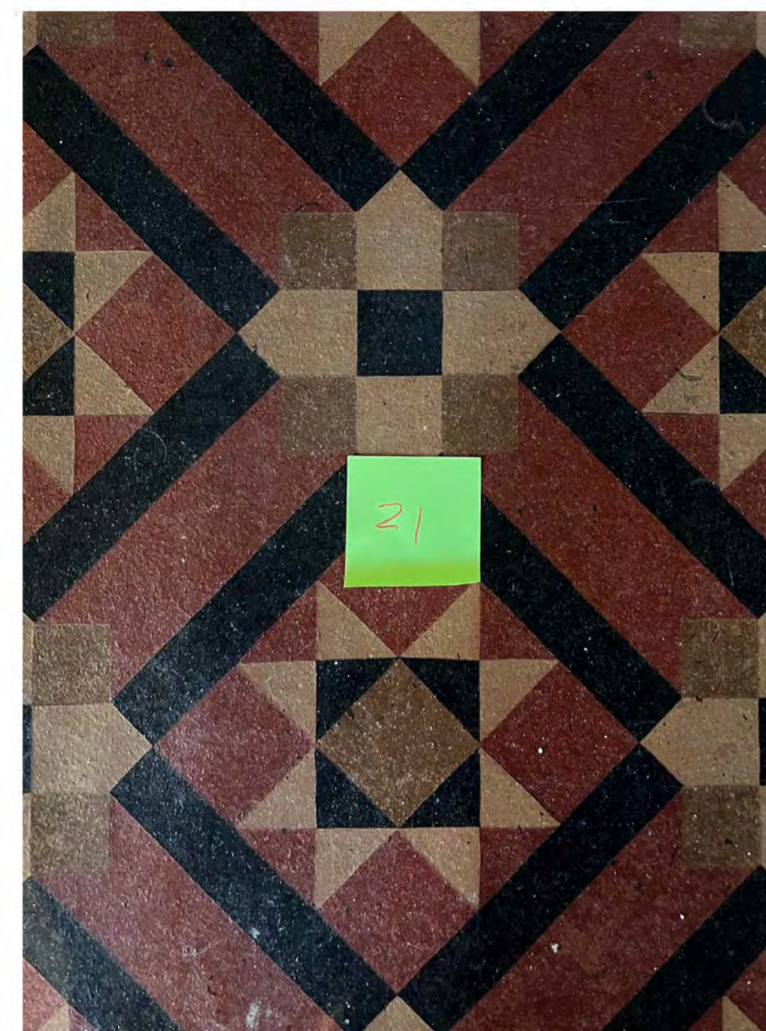
CODE: 1 CONDITION RATING: GOOD NUMBER: 21 GRID LOCATION: 3-DD
