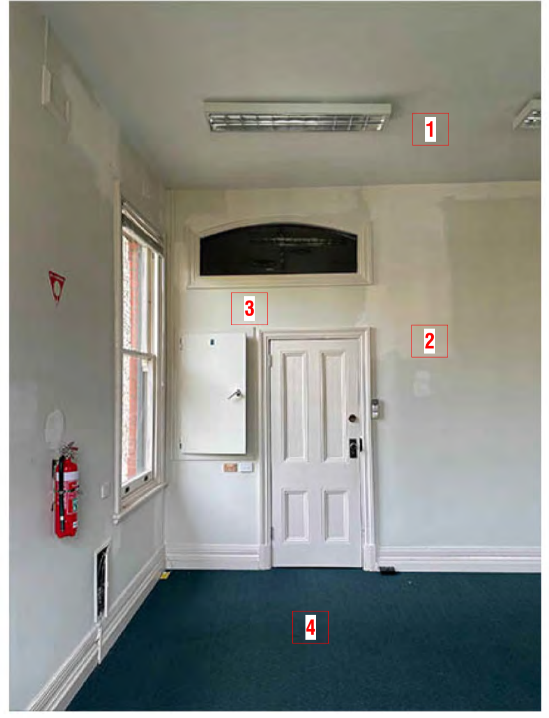
PHOTO - CURRENT VIEW OF ROOM WITH NON-ORIGINAL WALL
