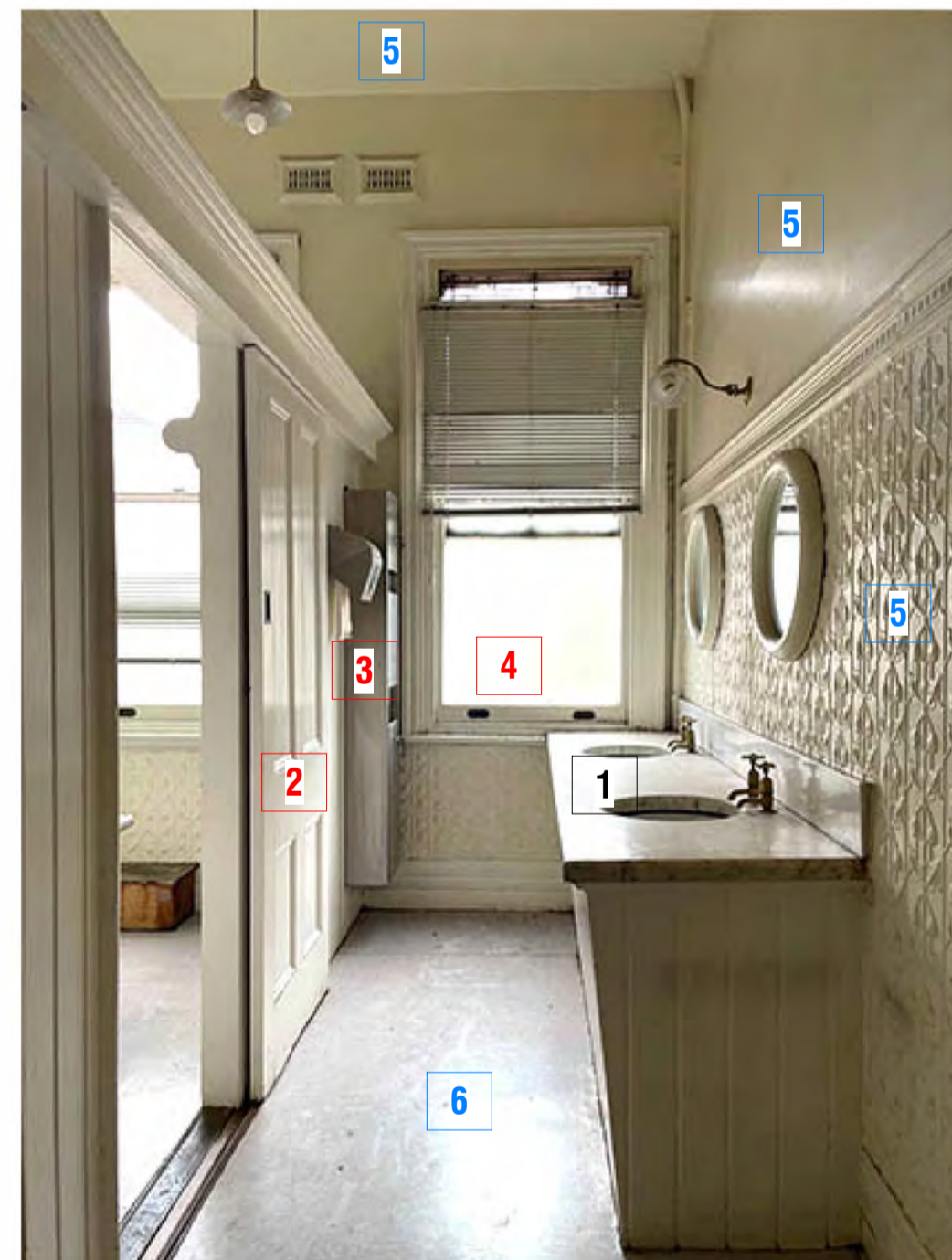
PHOTO - VIEW INTO CURRENT FIRST FLOOR BATHROOM
