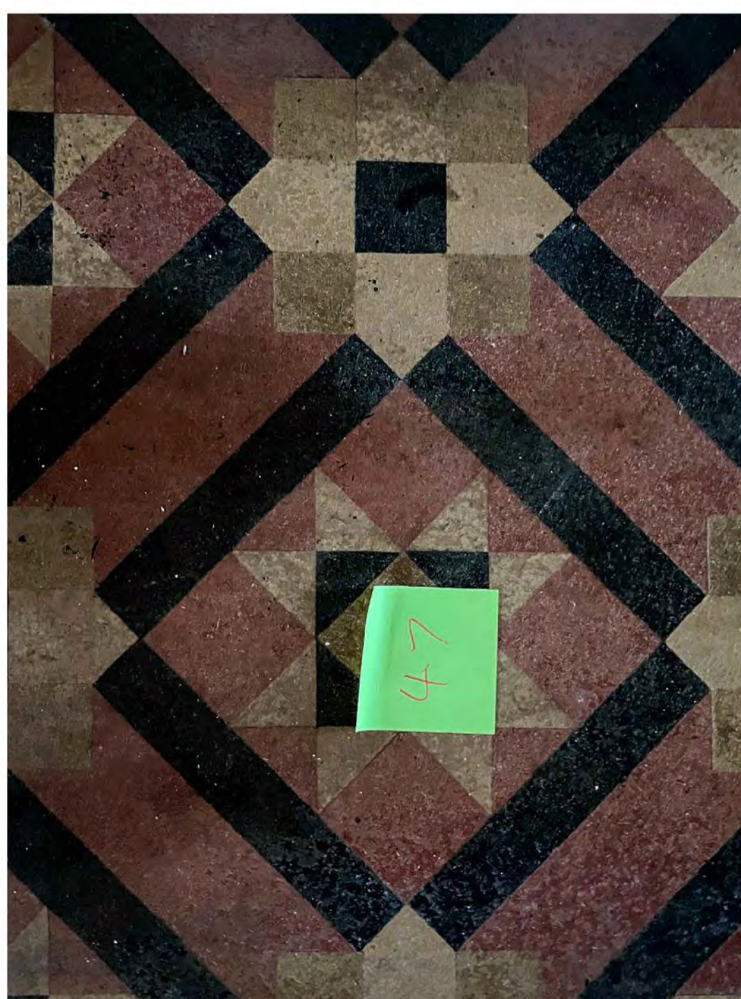
CODE: 1 CONDITION RATING: GOOD NUMBER: 47 GRID LOCATION: 5-AA
