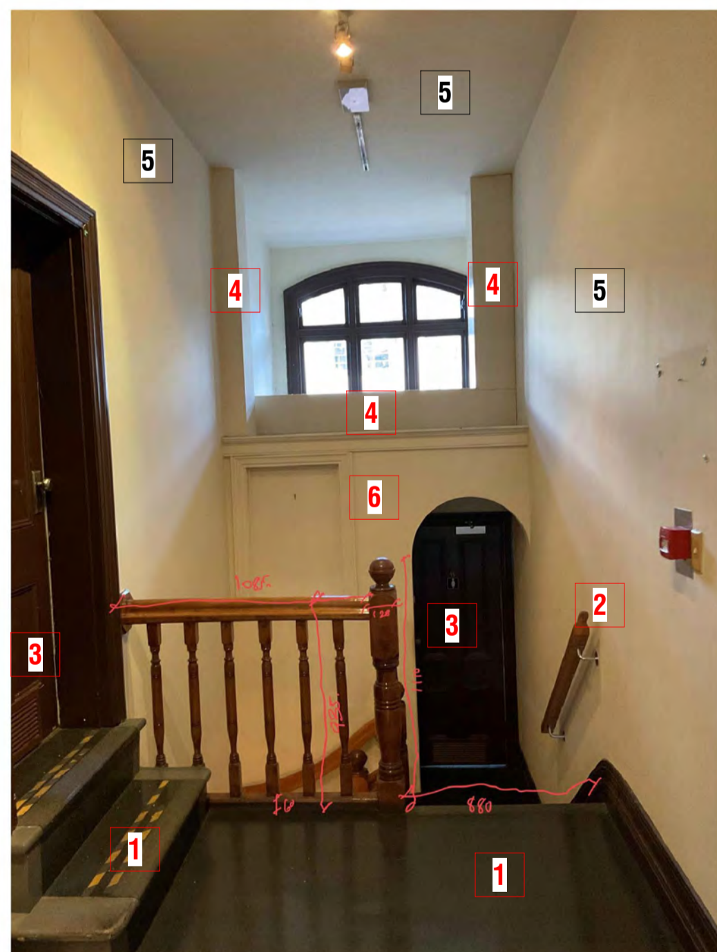
PHOTO - VIEW AT TOP OF CURRENT REAR STAIR LANDING
