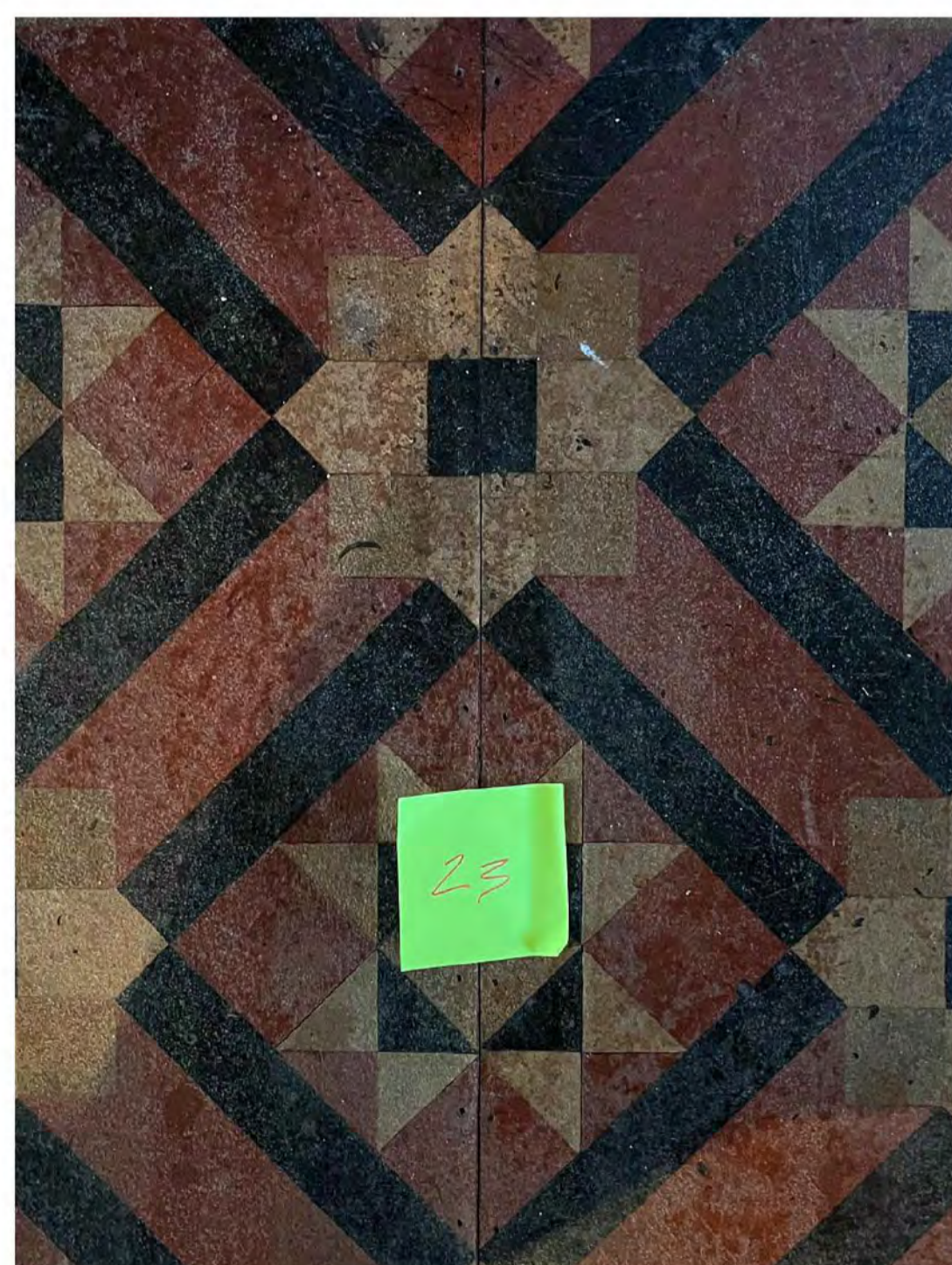
CODE: 1 CONDITION RATING: GOOD NUMBER: 23 GRID LOCATION: 3-DD
