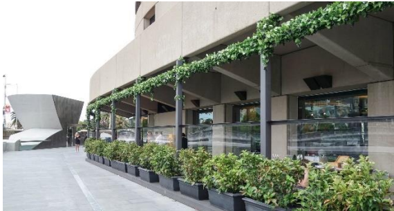
Figure 14 Image of exterior of Trocadero Restaurant with external steel frame structure, note current planter boxes not installed at this time, c.2013. Source: Dining Nirvana.
