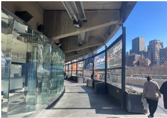
Figure 21 East end of the project area, not tapered beams to underside of upper terrace and later zig zag glazing to left of image. Source: Trethowan Architecture, 2024.
