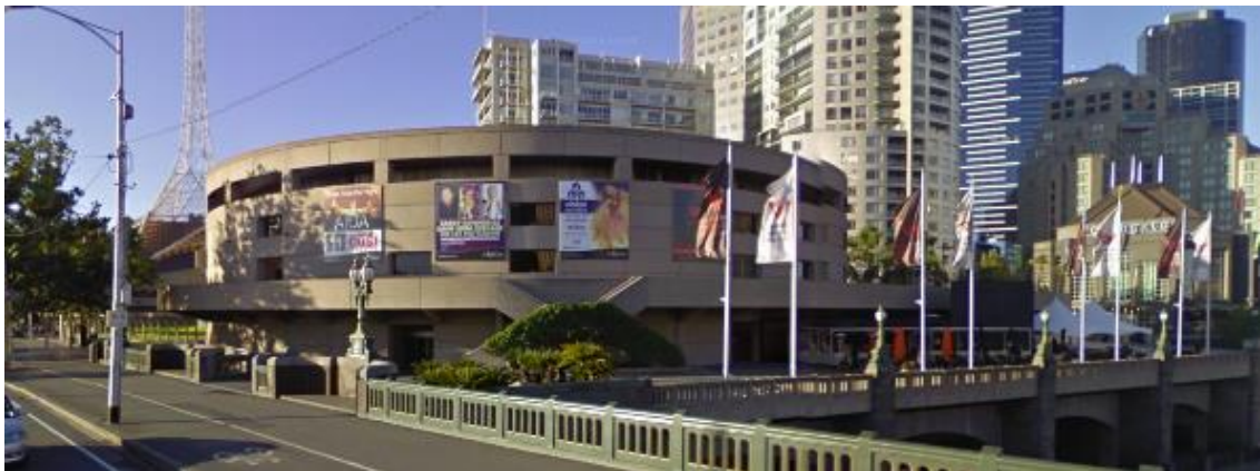
Figure 8 Hamer Hall in 2009 prior to redevelopment works. Note EQ Café and Bar and temporary promotional banners to the drum form. Source: Google Maps, 2009.
