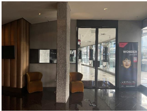
Figure 28 View into project area from Hamer Hall entrance foyer. Note, rectangular column with bush-hammered finish. Source: Trethowan Architecture, 2024.
