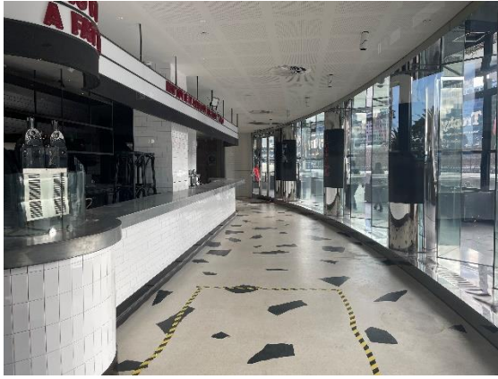
Figure 25 Interior of project area to east end. Note later terrazzo floor, bar and suspended ceiling from Fatto Bar & Cantina fit out. Source: Trethowan Architecture, 2024.
