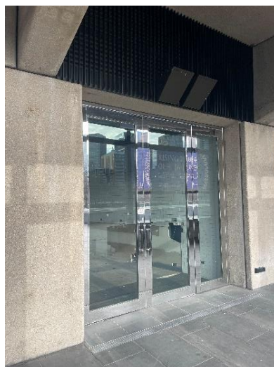
Figure 24 Later double doors with mirrored framing from the 2012 redevelopment works by ARM. Note also, ventilation grilles in dark bronze finish above door. Source: Trethowan Architecture, 2024.
