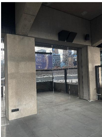
Figure 23 Later infill wall with mirrored panelling from the 2012 redevelopment works by ARM. Source: Trethowan Architecture, 2024.
