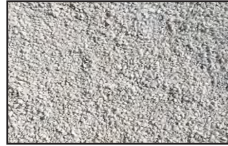
PV-02/A Compacted Gravel
