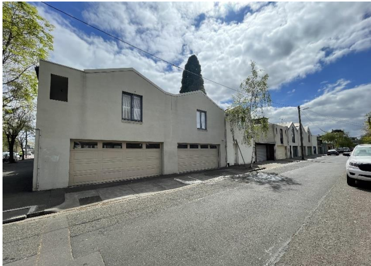
Figure 14, Bevan Street looking east from Montague Street (October 2023)
