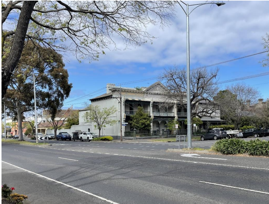
Figure 3, 1 St Vincents Place South existing conditions (October 2023)
