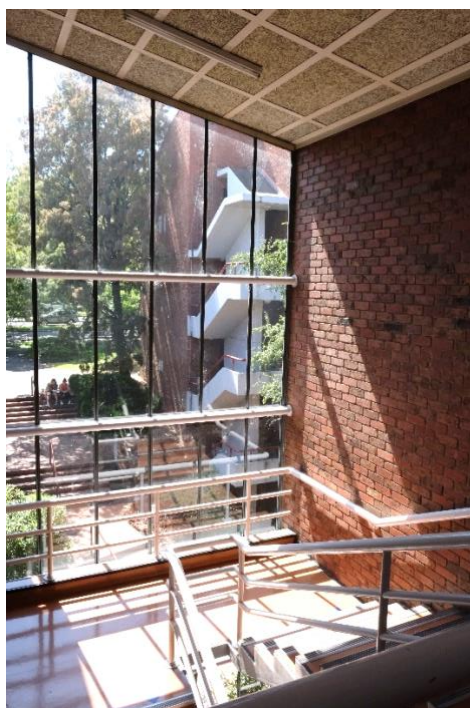
Figure 19 and 20. Internal stairwell (Source: GJM Heritage, January 2024)
