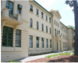
FORMER VICTORIA POLICE DEPOT SOHE 2008
