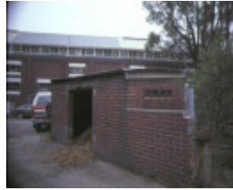
Former Victorian Police Mounted Branch Depot St Kilda Road Southbank Rear View March 1985
