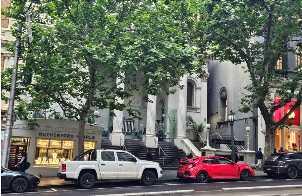
Figure 21: Image of the Collins Street Baptist Church, as viewed from Collins Street, facing north
