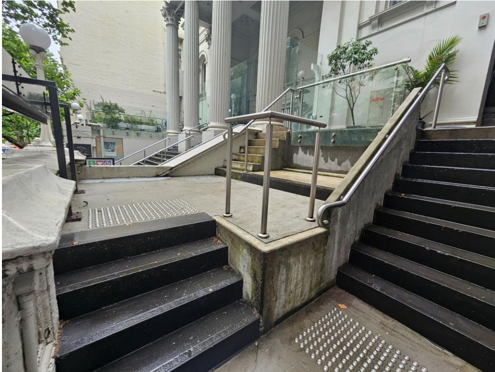
Figure 24: Image of the area to the southeastern corner of the Collins Street frontage, behind the low wall, facing west. The smaller of the bluestone stairs was introduced in 2010.
