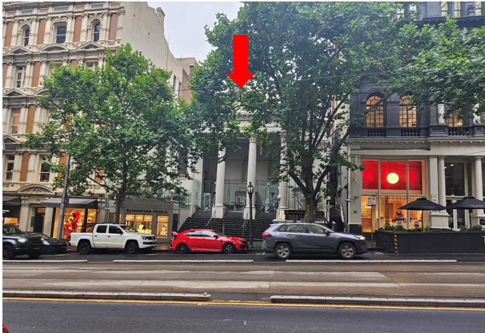
Figure 17: Image of the subject place (at centre and indicated by red arrow) showing the north side of Collins Street, facing north
