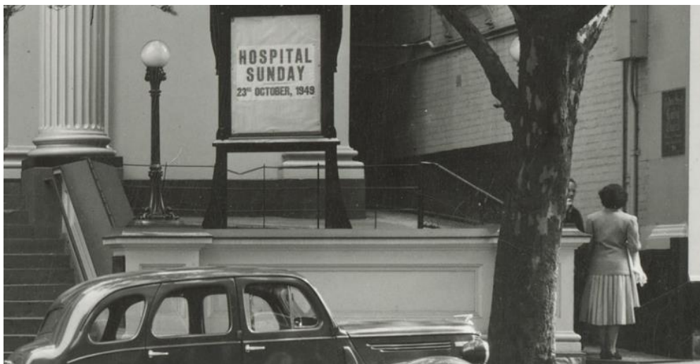
Figure 11: Close-up of late 1940s photograph of the Baptist church, showing the southeast corner of the Collins Street frontage (Source: SLV ID H2010.73/25)
