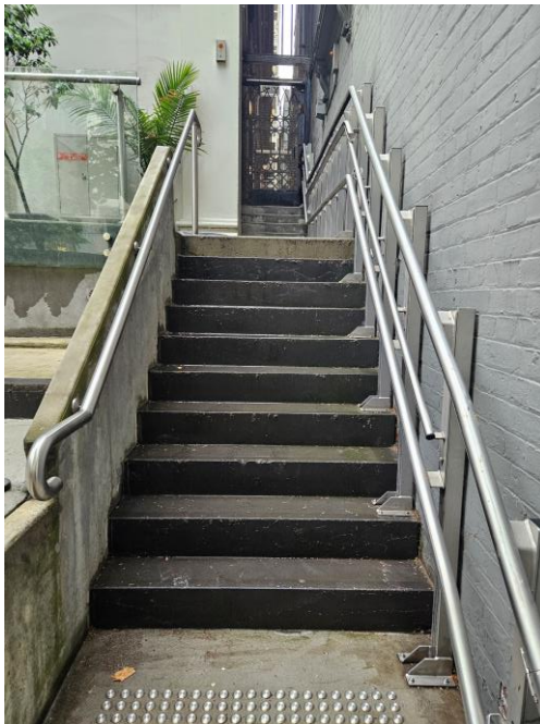
Figure 25: Image of the area to the southeastern corner showing the bluestone stairs leading from the lowest concrete landing to the topmost platform. The platform lift is visible to the right.
