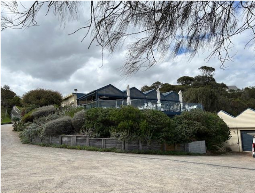
Photo: Photo taken from the Clubhouse carparking. No views of the extension can be seen from this view. Parts of this building will remain the same.
