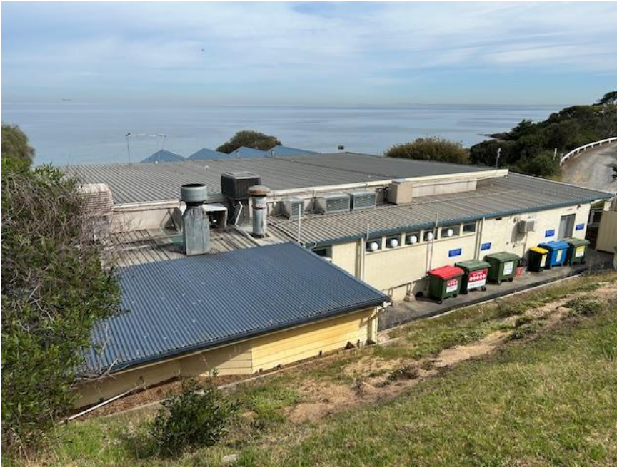
Photo: Photo taken from the top of the embankment. Roof line of the building lower than the embankment. Blue roof building at the forefront is to be demolished for the new extension.
