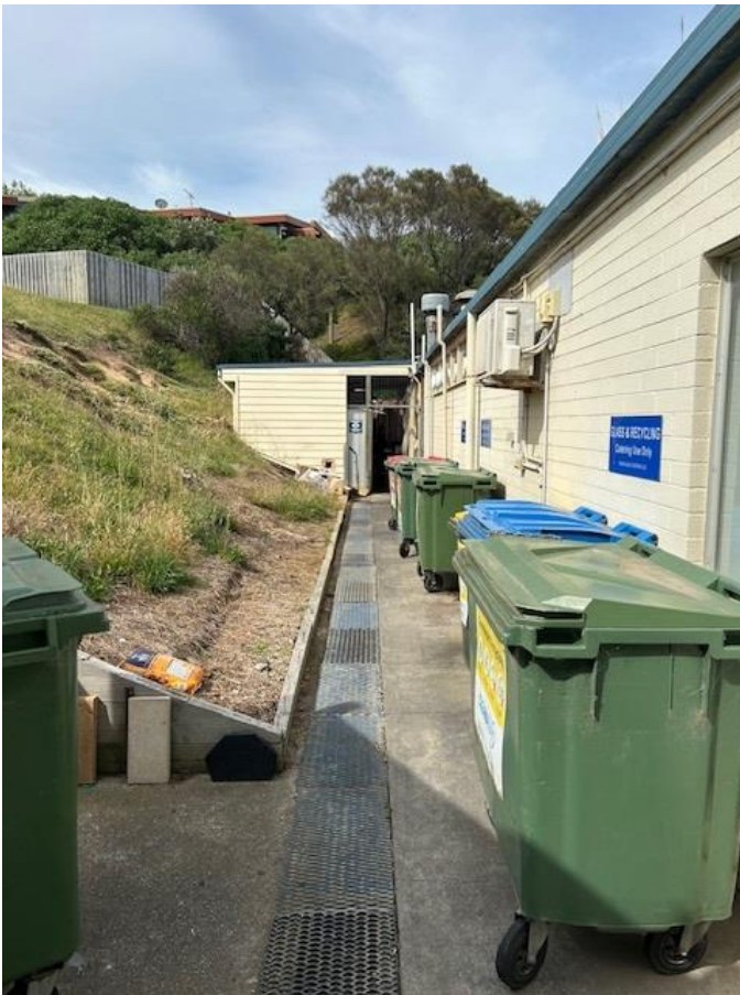
Photo: Photo taken at the rear of the Clubhouse. Extension of the building will be seen at this level with demolition of the outbuilding.
