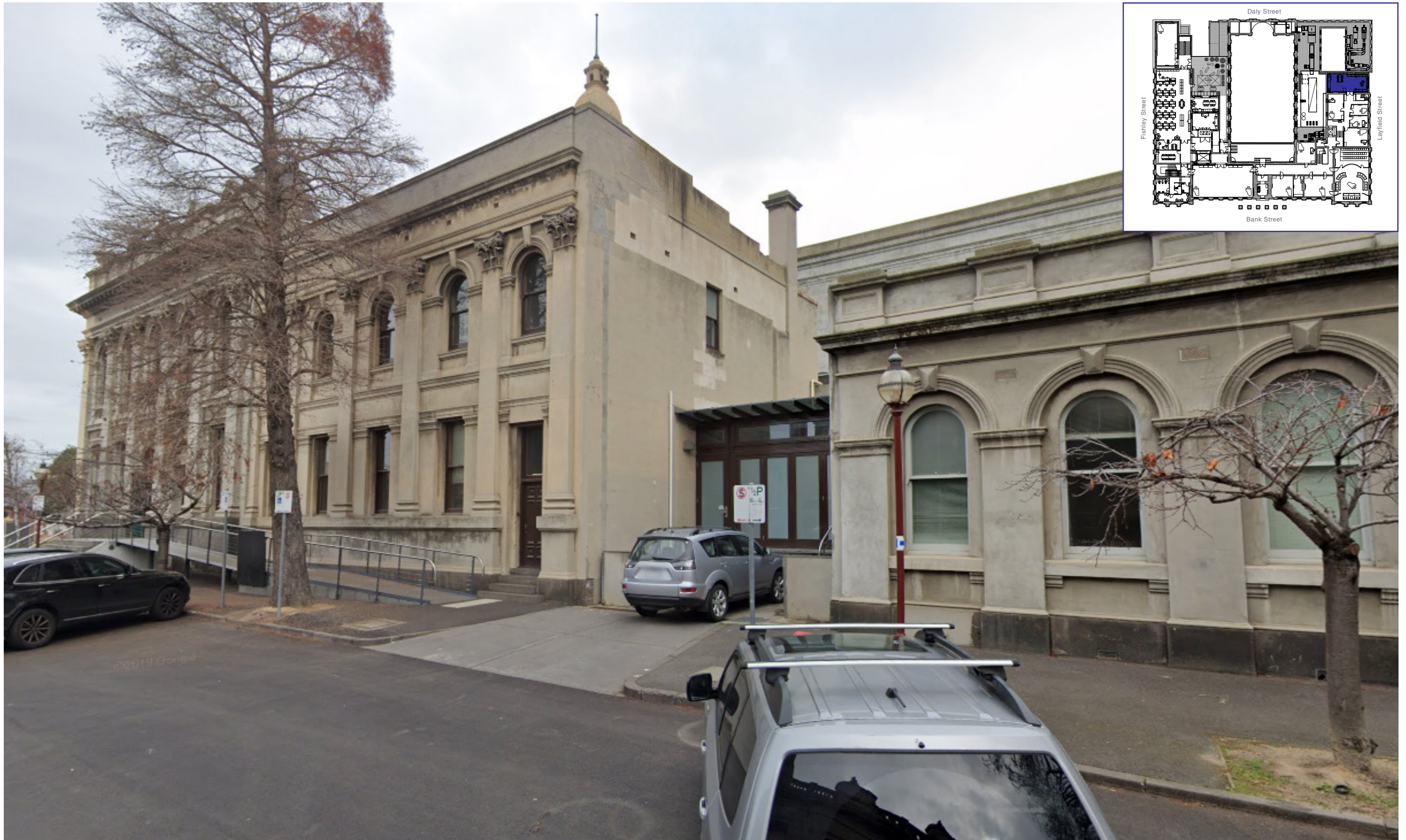
Layfield St Frontage - Google Street View (Winter 2019)
