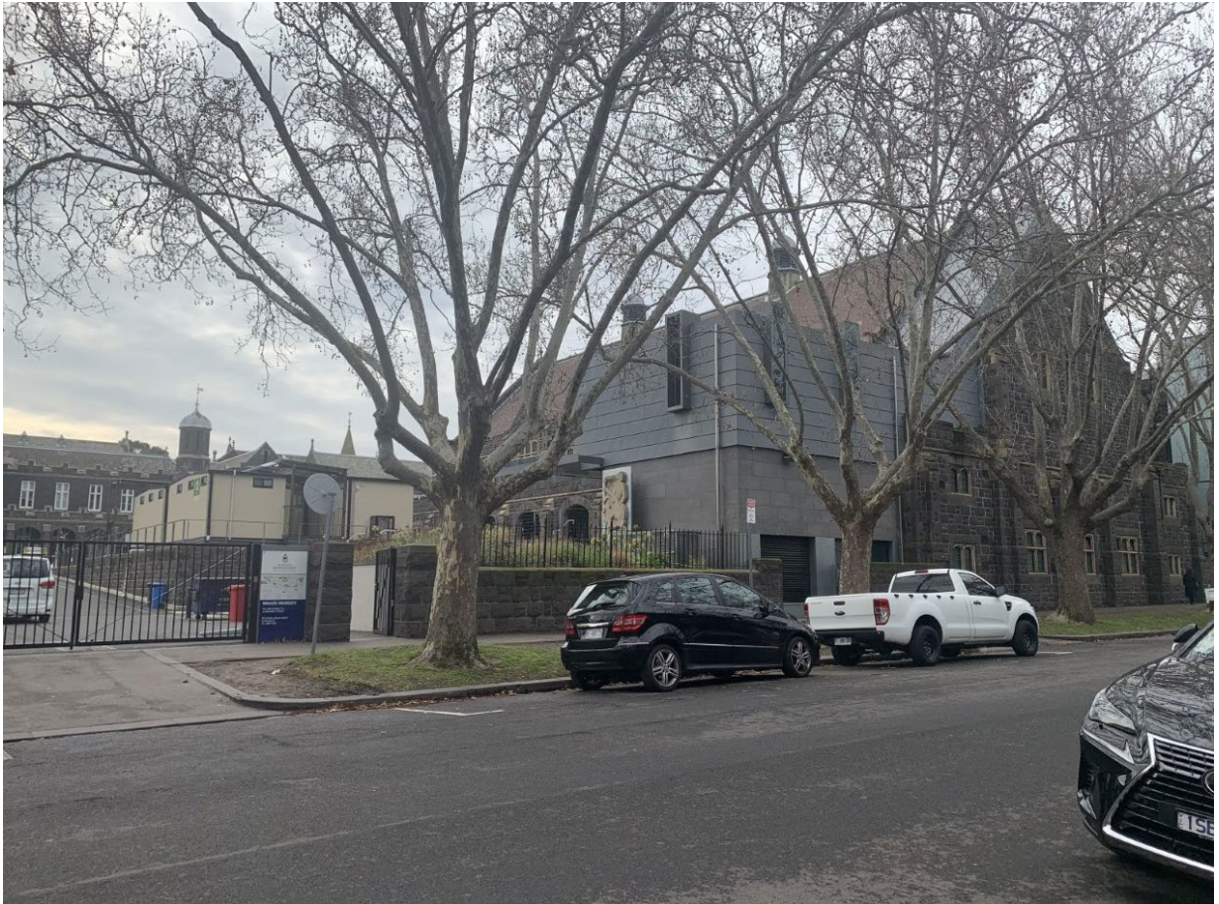
Figure 8 - Existing Site Conditions (Bromby Street - Opposite Streetside View)
