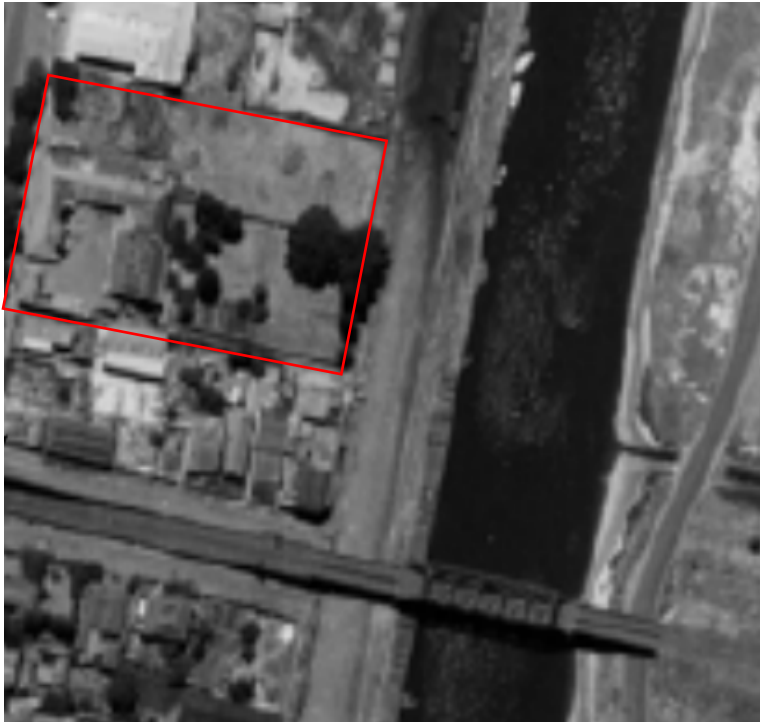
Figure 13 The study area in 1951 (Land Information Office of the Department of Sustainability and Environment, 2023)
