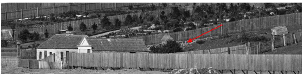
Figure 5 The river section and Moreland Street section of the study area with bluestone retaining wall, 1875 (Mitchell Library, state Library of New South Wales)
