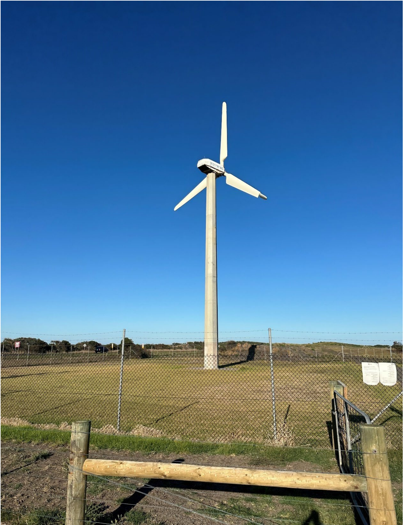
Figure 3 Another view of the turbine, from Blackrock Road looking east Source: Lovell Chen, 2025
