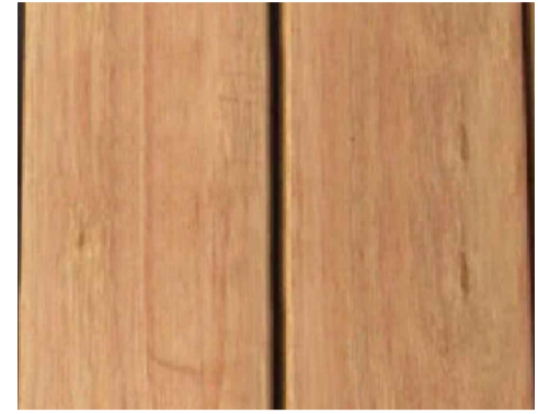
DECKING - MERBAU BLANKBUTT OTHERWISE TO MATCH EXISTING.
